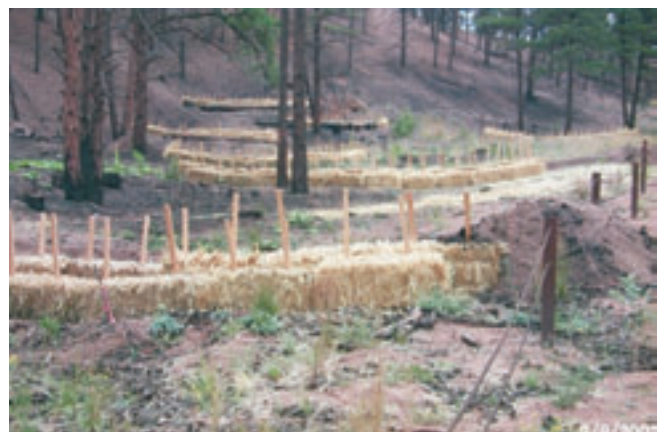
Figure 14 —Straw bale check dams on Denver Water Board property within the Hayman Fire area.
