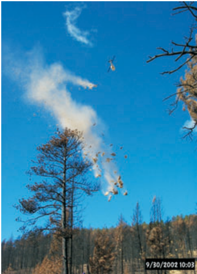
Figure 11 —Aerial dry mulch being applied.
