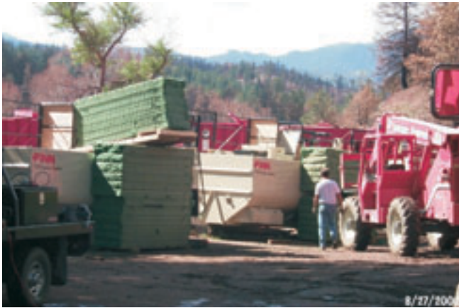
Figure 7 —Aerial hydromulch staging area.
