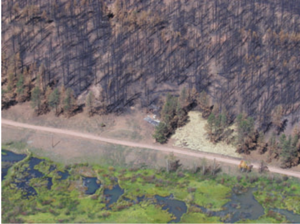
Figure 25 —Aerial photograph of a home in Lost Valley Ranch designated as destroyed by torching/crown fire. Note the unburned vegetation immediately adjacent to the home on the right as well as other unburned vegetation.
