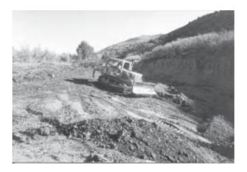
**Figure 36**—Three-way dozer reshaping a streambank.
