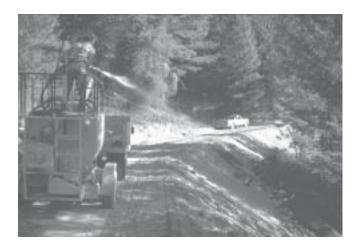
Figure 33—Hydroseeding roadcuts and fills.
