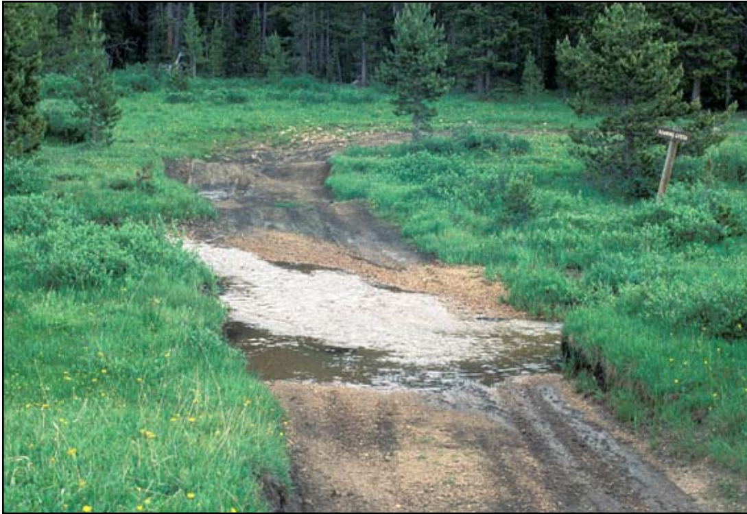
Figure 14. Forest roads can degrade stream habitats by serving as a chronic source of fine sediment, as well as providing access points for illegal introductions of nonnative species. This stream ford is immediately upstream from a key spawning area for Colorado River cutthroat trout (although it is in a river basin historically supporting greenback cutthroat trout). Roaring Creek, Colorado.
