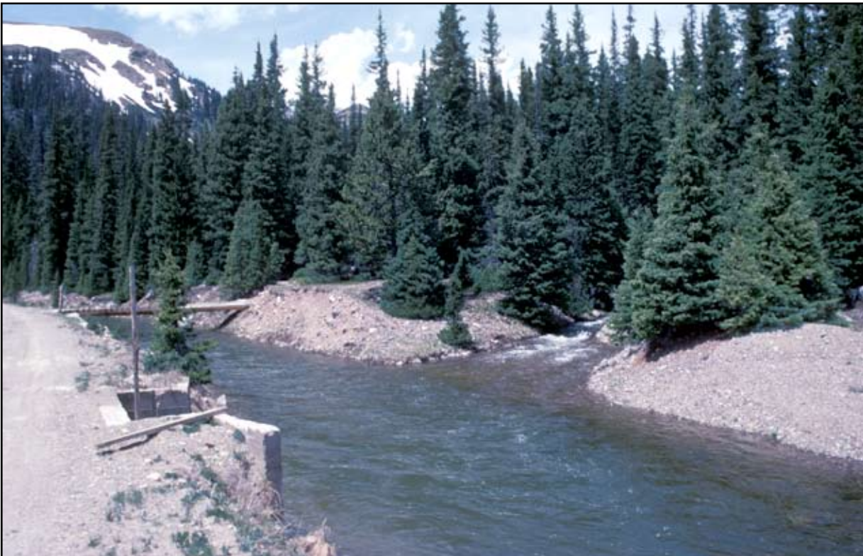
Figure 15. The Grand Ditch, built in 1890, reroutes water from the upper Colorado River basin into the Cache la Poudre River on the east side of the Continental Divide. As well as reducing streamflows in the Colorado River in Rocky Mountain National Park for over a century, it may have served as one of the initial conduits for the invasion of Colorado River cutthroat trout into waters historically occupied by greenback cutthroat trout.
