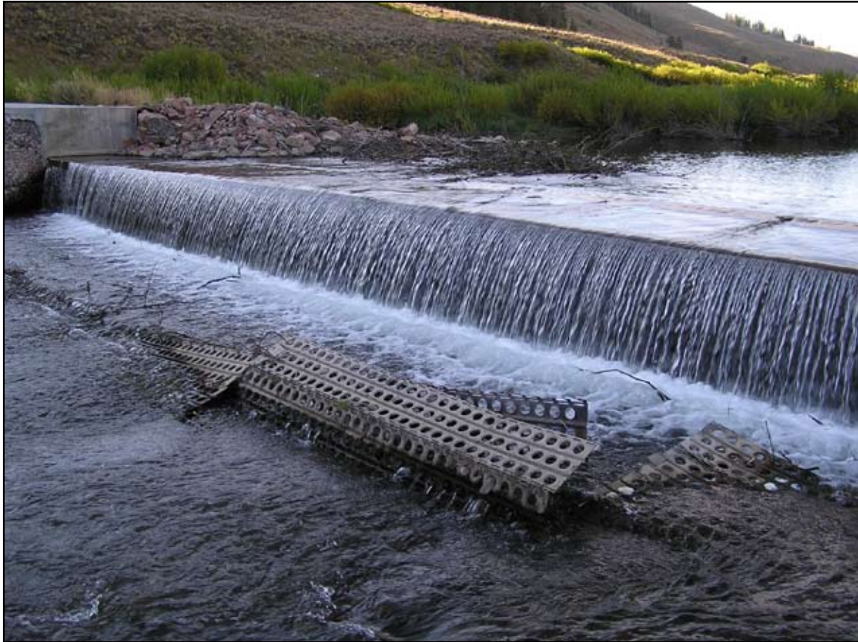
Figure 18. Artificial barriers are designed to prevent upstream migrations of nonnative fish species, but these structures require regular maintenance to remain effective. LaBarge Creek, Wyoming.
