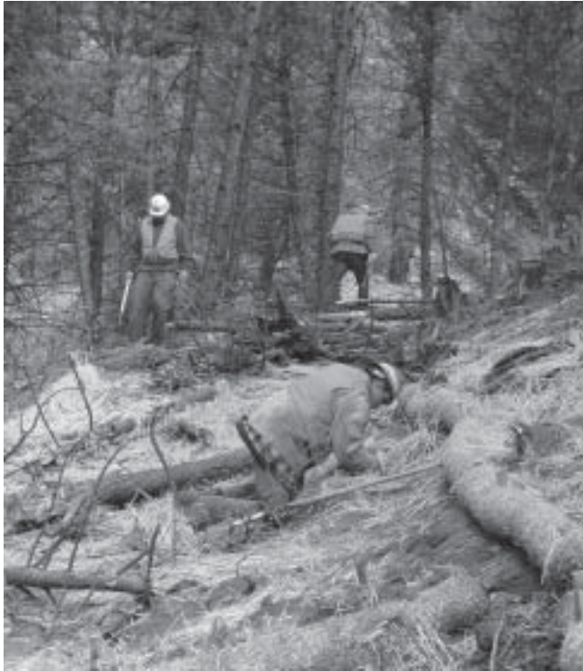
Figure 5 —Revegetation of access roads, Bitterroot NF (photo by Craig Odegard).
