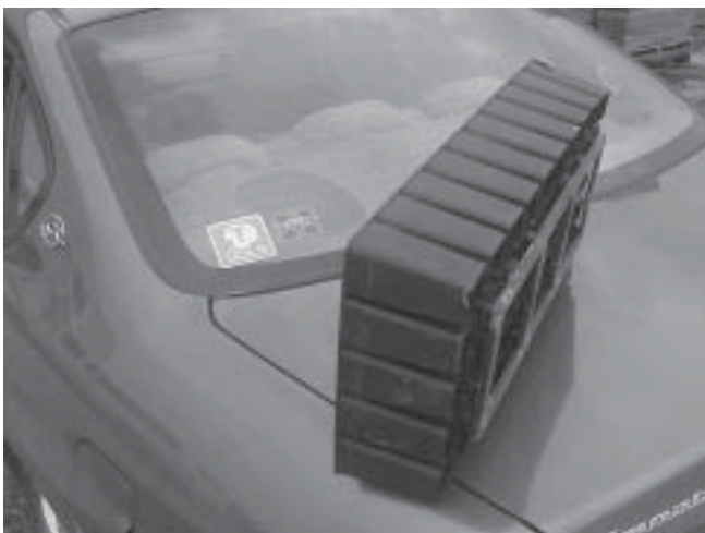
Figure 2 —“Vic Pot” 50 cavity tray with drip rail.
