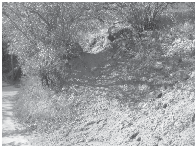
Figure 2 —Damage and erosion caused by heavy off-trail use by visitors.
