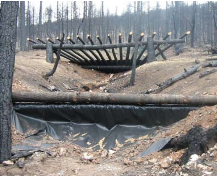
Trash rack and silt dam before (above) and after (right) first thundershower following fire.
