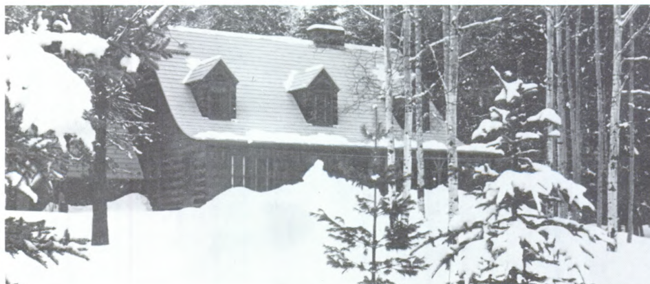
Figure 4.—Ice usually accumulates at the edge of overhanging eaves of heated buildings (photographed March 12, 1964).
