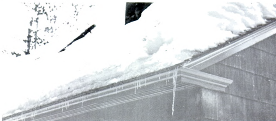
Figure 4.—Ice usually accumulates at the edge of overhanging eaves of heated buildings (photographed March 12, 1964).
