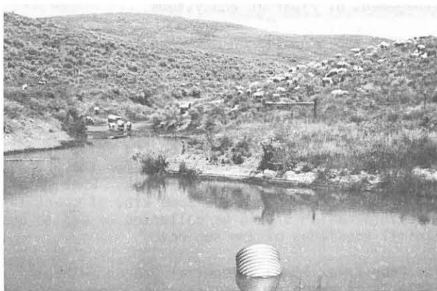
Figure 1.--An effective check dam in a 7-ft deep channel.
