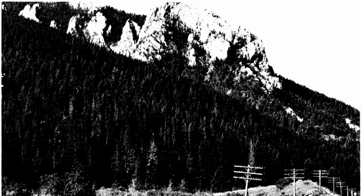
Plate 77b (July 19, 1981) About 77 years later A long period free of disturbance has allowed development of a dense stand of Douglas-fir mixed with lodgepole pine. Photograph by R. F. Wall.
