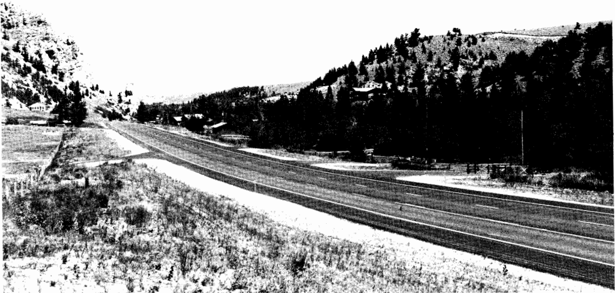
Plate 81b (July 8, 1981) 60 years later Camera point was moved across U.S. Highway 212 in order to avoid trees which screened original view. Deciduous vegetation along stream course is being replaced by Douglas-fir and spruce, while slopes in distance at left and beyond Rock Creek show a significant increase in density of limber pine. Photograph by R. F. Wall.
