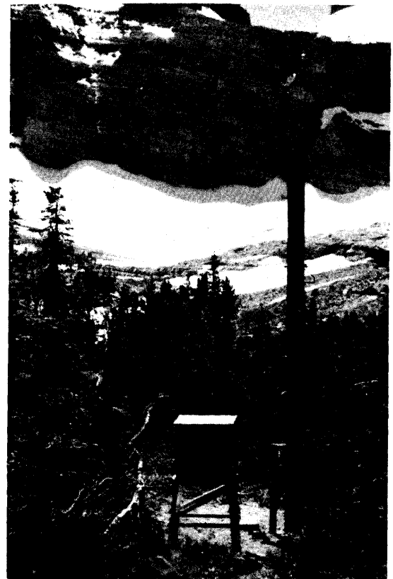
Figure 12.—Storage precipitation gauge (21-ft standpipe) and thermometer shelter near Grinnell Glacier (site No. 1, averaging 100-inch [2 540-mm] annual catch), July 1960.
