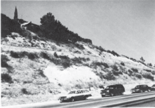
Figure 3 —The same road cut 10 years after a more expensive, more complicated, but less successful attempt at restoration.
