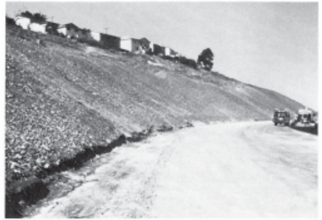
Figure 1 —A 1 1/2:1 road cut restored using a low-cost but technically adequate concept.
