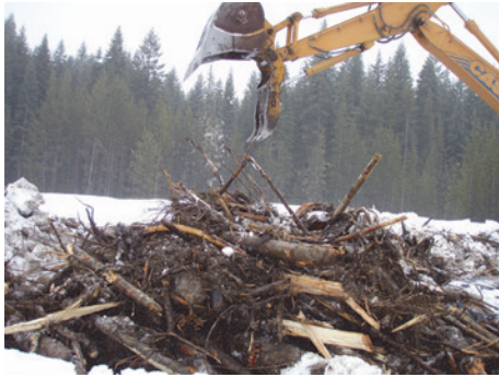
FIGURE 1: Elevated machine pile being constructed. (Photo credit: J. G. Archuleta.)
