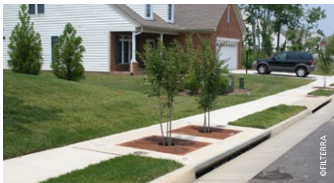
Linear stormwater tree pit
