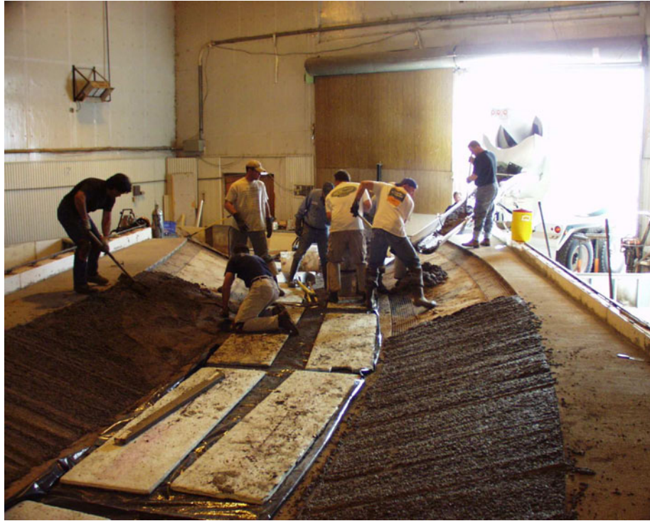
Figure A.9 Concrete Placement for Model Construction
