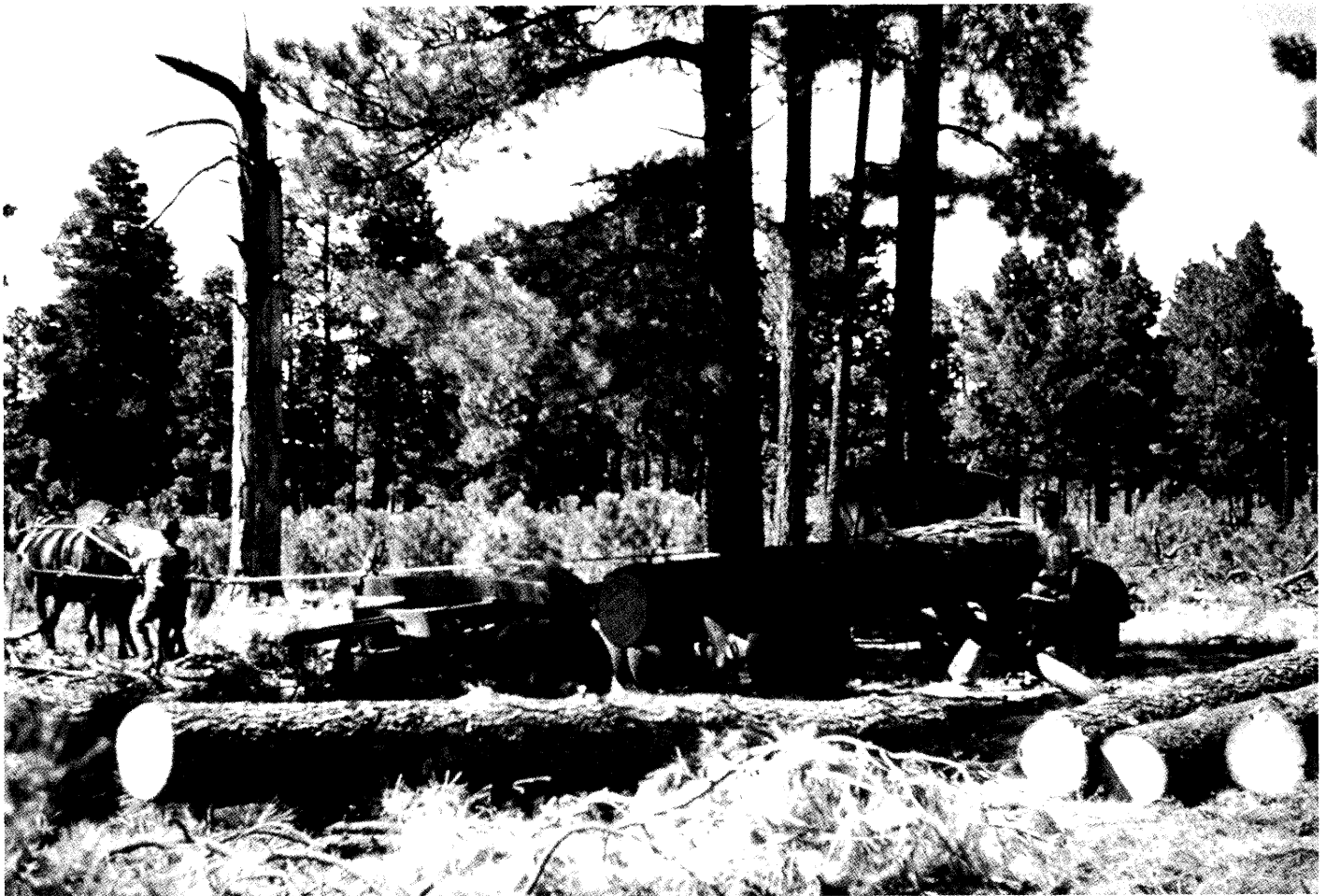
Figure 8.2 Even large-sized material can be handled with horse and small-equipment; these heritage methods may still be useful for operating at low cost and without damage to the soil and residual trees.
