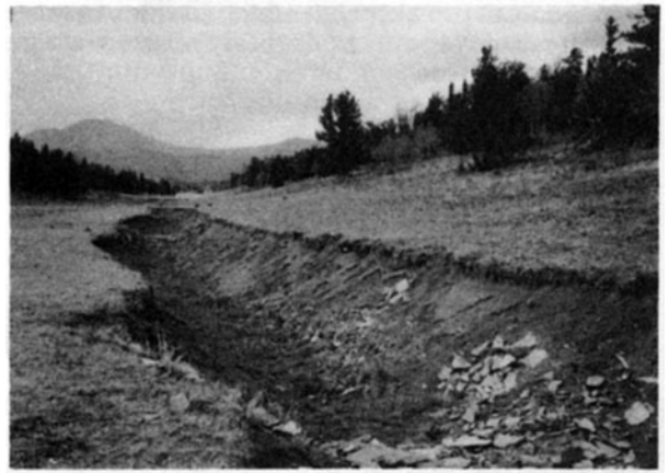
Figure 13.—Erosion channel through a Front Range meadow.
