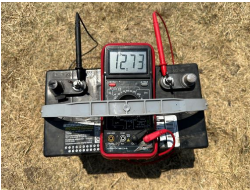
Figure 13 Fully charged battery.
