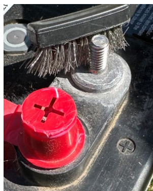
Figure 16 A battery being cleaned of corrosion with a metal bristle brush.
