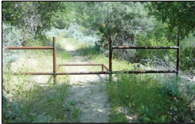
Figure 3—A horse stile. This gate is not accessible because the bars across the opening are higher than 1 inch.
