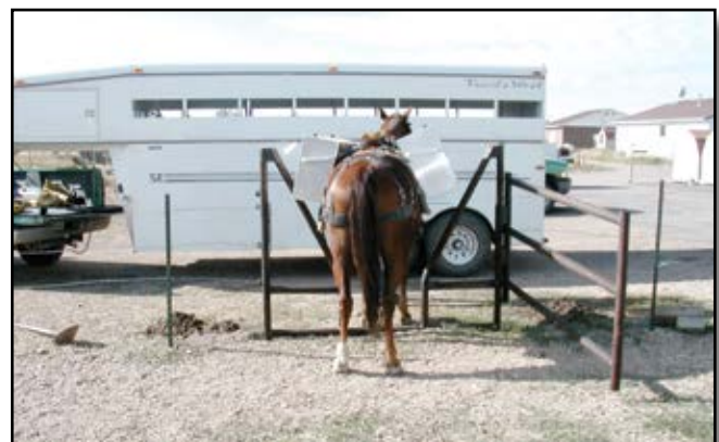
Figure 1—A horse walking through a “V” gate in Utah. This gate is not accessible because it is narrower than the minimum width required for passage of a wheelchair (36 inches) and the bar across the opening is higher than 1 inch.
