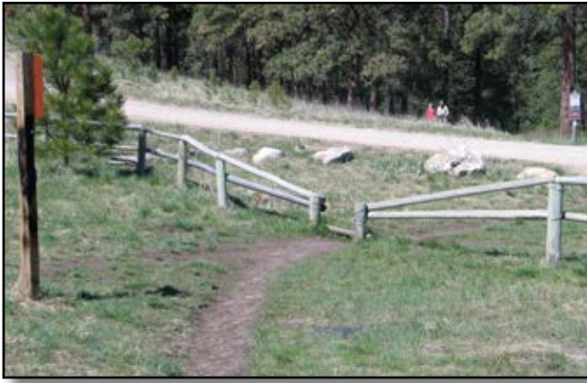
Figure 2—A gate in the Lolo National Forest that allows horses to pass, but restricts ATVs. This gate is not accessible because it is narrower than the minimum width required for passage of a wheelchair (36 inches) and the bar across the opening is higher than 1 inch.
