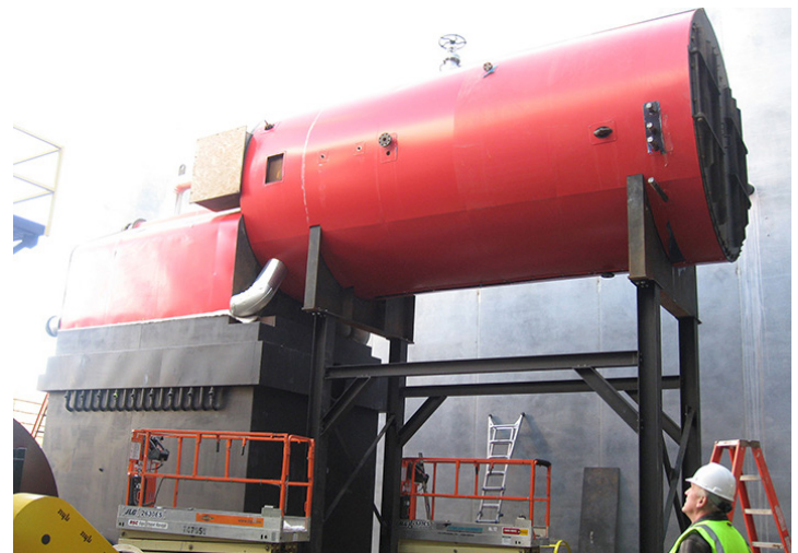
This biomass boiler is one part of Gundersen Health System's sustainable power generation. Courtesy photo by Gundersen Health System.
