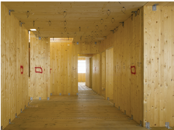
Stadthaus interior during assembly (CLT panels), Murray Grove, London, England Used by permission of Will Pryce
