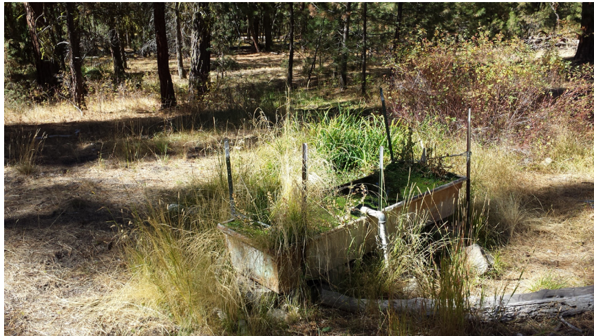
Figure 11. A development needing rehabilitation. Overflow from the trough does not return to the spring ecosystem, wasting a valuable resource in a dry landscape and depriving aquatic fauna (spring snails) of habitat. (Photo courtesy of The Nature Conservancy.)
