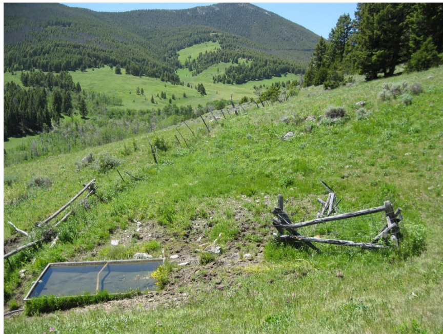
Figure 1. Example of a poorly designed and maintained spring development. Lack of valves results in continuous flow and desiccation of the spring habitat. Trough is in the spring source area causing trampling of organic soils. Enclosure fence is nonfunctional. (Photo by USDA Forest Service.)
