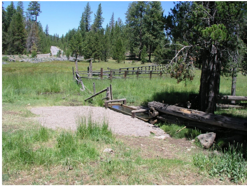
Figure 12. A well designed but poorly maintained spring development. A gravel-hardened surface next to the trough prevents erosion and sediment and the low elevation trough allows access for wildlife. Note: Enclosure fence around important wetland area is in disrepair. (Photo by USDA Forest Service.)
