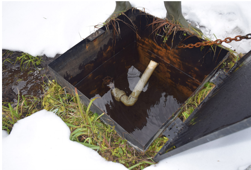
Figure 5. View of the interior of the spring box at a diffuse discharge spring. The elbow joint is adjustable and is set to maintain the threshold water table depth determined for the spring and the season. (Photo courtesy of The Nature Conservancy.)
