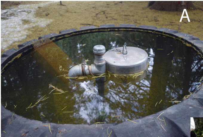
Figure 10a. Tractor tire trough at a spring. A large float valve like this resists damage from cattle. (Photo courtesy of The Nature Conservancy.)
