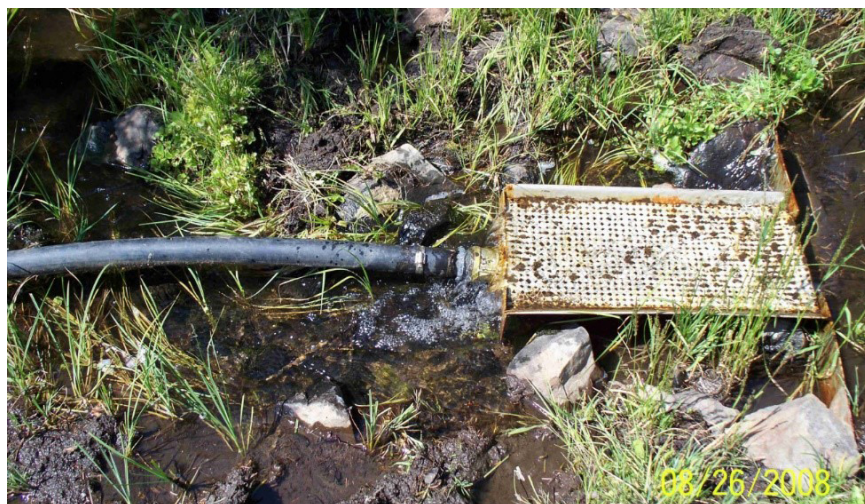
Figure 9. Pipeline collection tray in a spring channel. (Photo by USDA Forest Service.)
