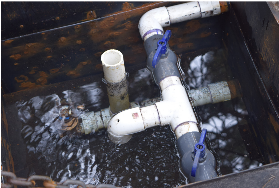
Figure 7. Valves control the flow of water at this spring box. There is always some water routed to the spring to keep the ecosystem functioning. The trough is fitted with a float valve so water is diverted from the spring only when a demand is present. (Photo courtesy of The Nature Conservancy.)
