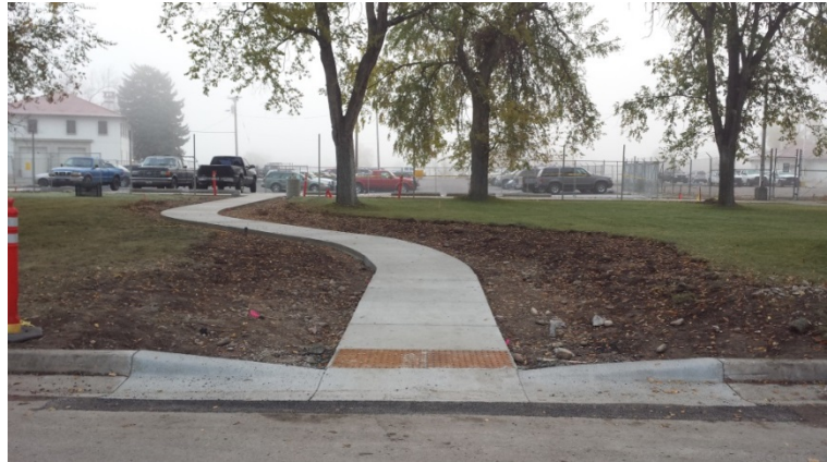
New ADA compliant sidewalk has been installed.
