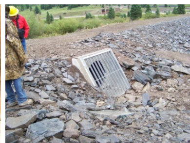
After: New emergency spillway.
