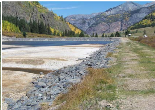
After: The dam is now safer. It has an operable outlet and emergency spillway. It has protection from wind erosion with placed riprap and the vegetation clearing allows seepage to be more visible to quantify and correct.
