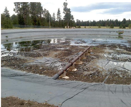
Failed Liner before start of project.
