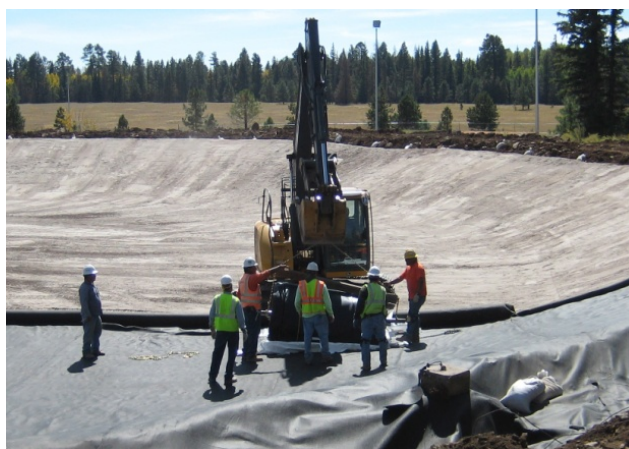
Lagoon at the beginning of the installation of new Polyolefin Liner. Project was completed at the end of FY 2012.
