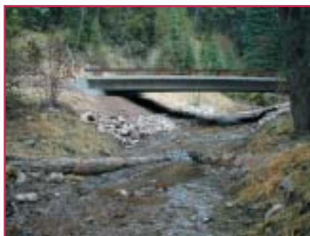
Figure 4 —Large-span bridge installed to replace a degraded culvert as part of the Clearwater Project on the Seeley Lake Ranger District. For the first time in many years, spawning bull trout could pass upstream from the bridge. Photo: USDA Forest Service.
