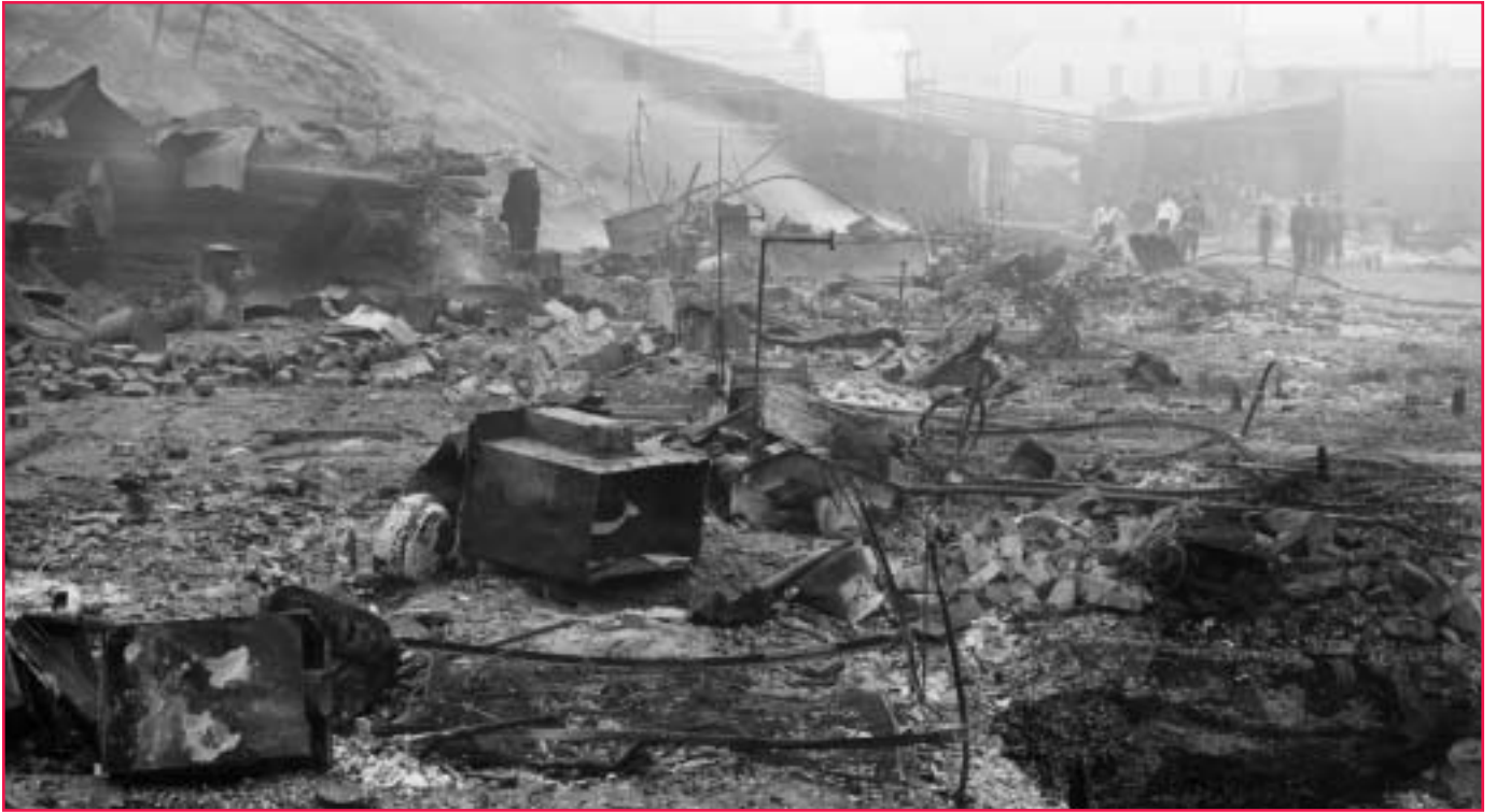
Destruction at the eastern end of Wallace, ID, following the Big Blowup of 1910. Photo: Courtesy of the Barnard-Stockbridge Collection (8-X0545d), University of Idaho, Archives and Special Collections.
