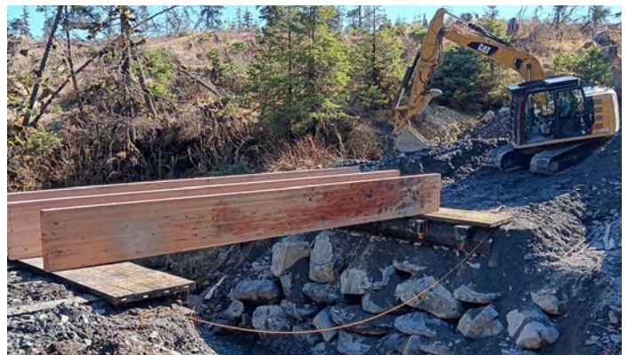
Installing a Koniag temporary bridge. Image courtesy of Peter C. Olsen.
