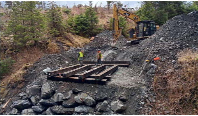
Preparing the site for a Koniag temporary bridge. Image courtesy of Peter C. Olsen.
