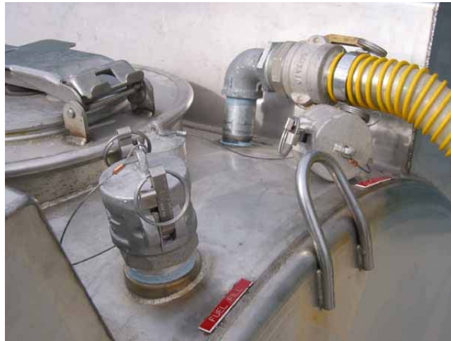
Fill and Vapor Connections Fill Connection in Foreground
