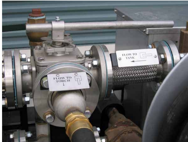
Directional Control Valve Handle in “Flow to Tank” Position
