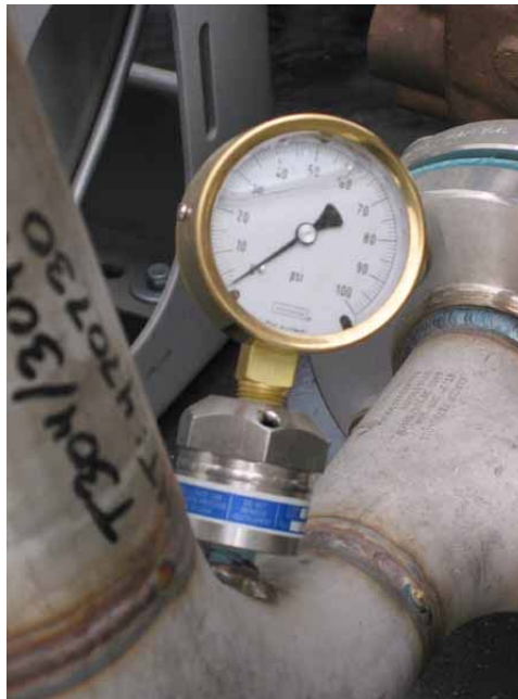
Gage and Diaphragm Assembly
