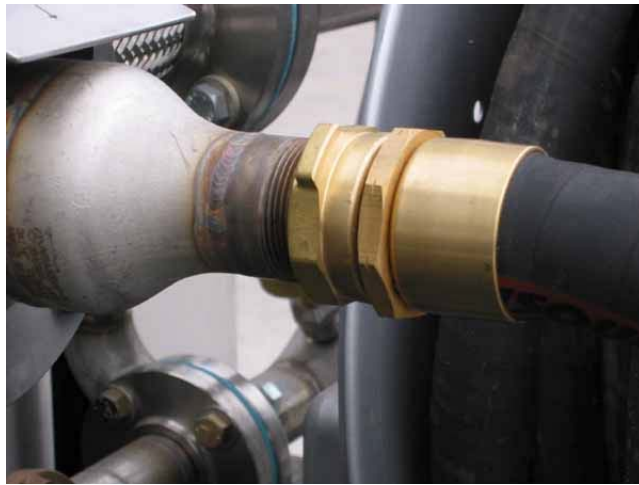
Directional Valve Hose Connection
