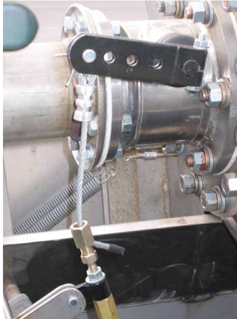
Tank Re-circulation Valve Fusible Link and Cable
