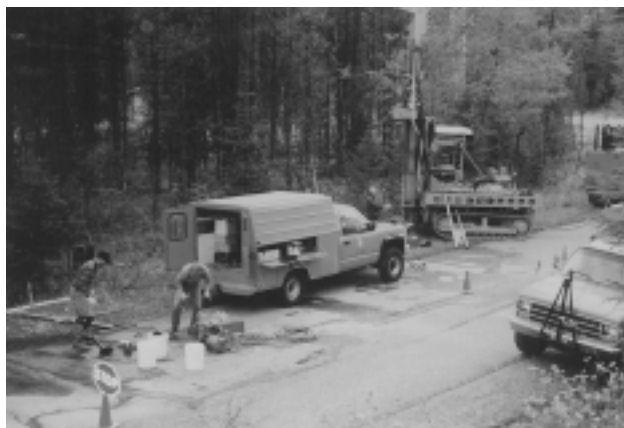
Figure 44—Kootenai National Forest—Site 1 during instrumentation installation.
