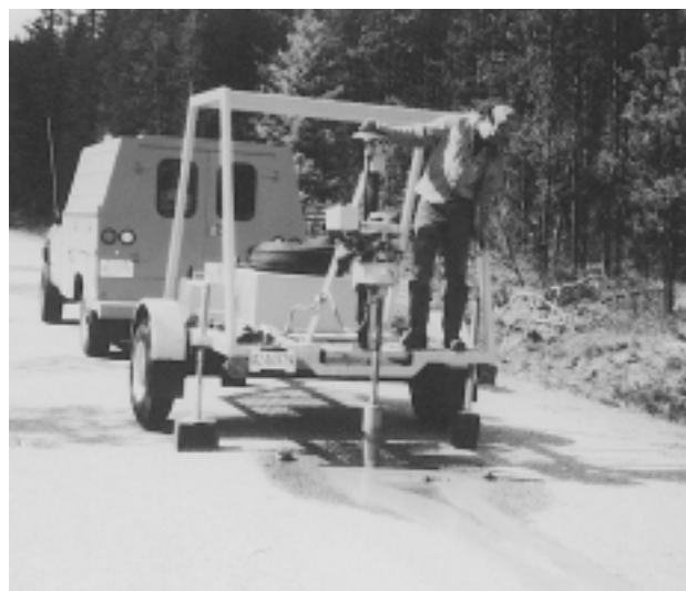
Figure 49a—Drilling AC pavement cores for laboratory modulus testing. Kootenai National Forest—Site 2.
