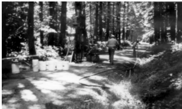
Figure 16—Willamette National Forest test site during instrumentation installation. The narrow, aggregate surfaced road is typical of many western Oregon FS roads.
