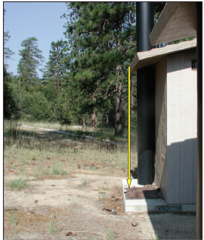
Figure 1—The roof dripline is directly over the manhole in the single vault CXT toilet building.
