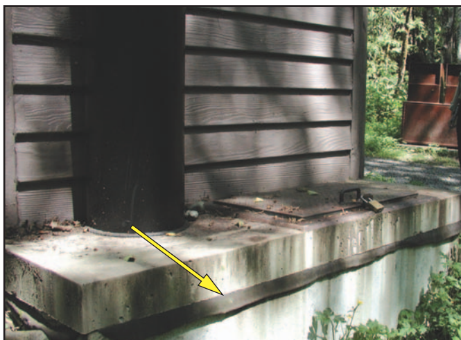
Figure 5—Mastic between the vault and building slab make a watertight seal
