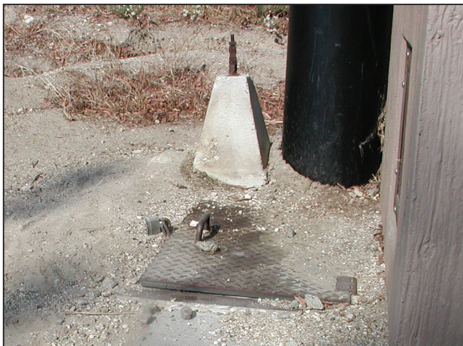
Figure 3—Debris under gasket.
