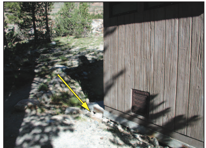
Figure 6—This vault is below finished grade. The mastic between the building slab and vault is damaged. The vault fills with water every spring.
