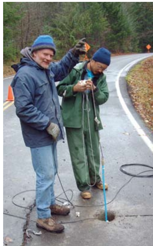
Figure 2—Installation of TDR coaxial cable into auger hole.
