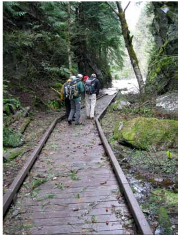
Figure 2—Forest Service Region 6 Iron Goat Trail, made of 100 percent HDPE RPL, installed in 2004.
