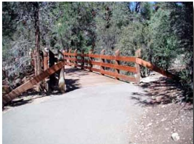
Figure 9—Bridge made of Ipe wood.
