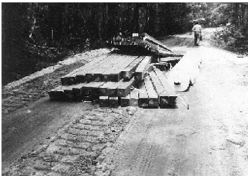
Figure 4. Geotextile and mats ready for installation.
