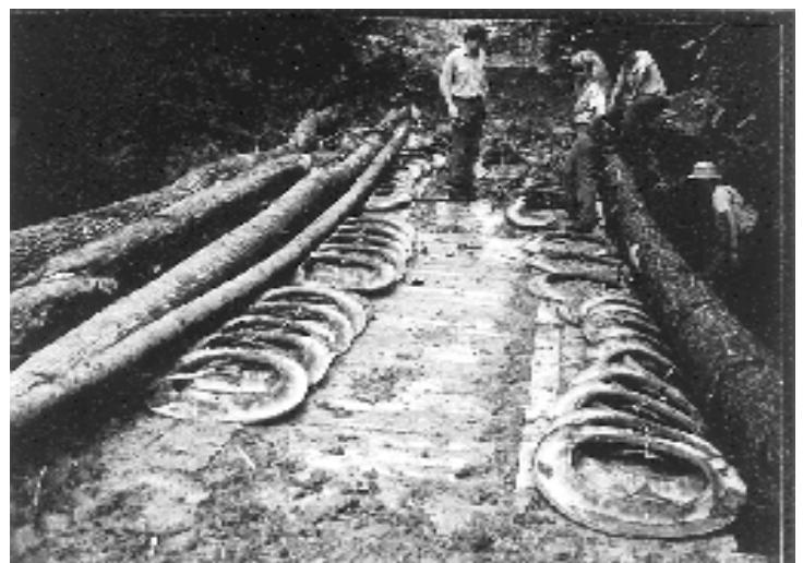
Figure 9. Deterioration of Terra Mat from skidding logs.
