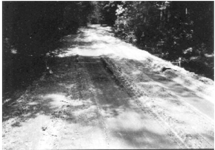
Figure 2. Ruts in road prior to placement of portable crossing.
