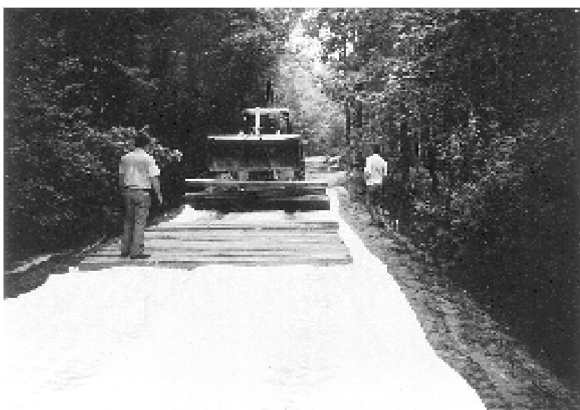
Figure 5. Wood mat and geotextile installation in progress.
