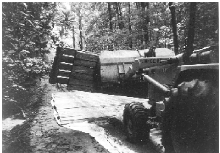
Figure 3. Placement of pallet sections.
