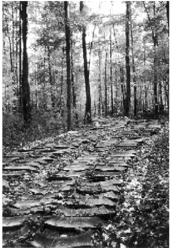
Figure 6. Terra Mat constructed of tied together tire sidewalls.
