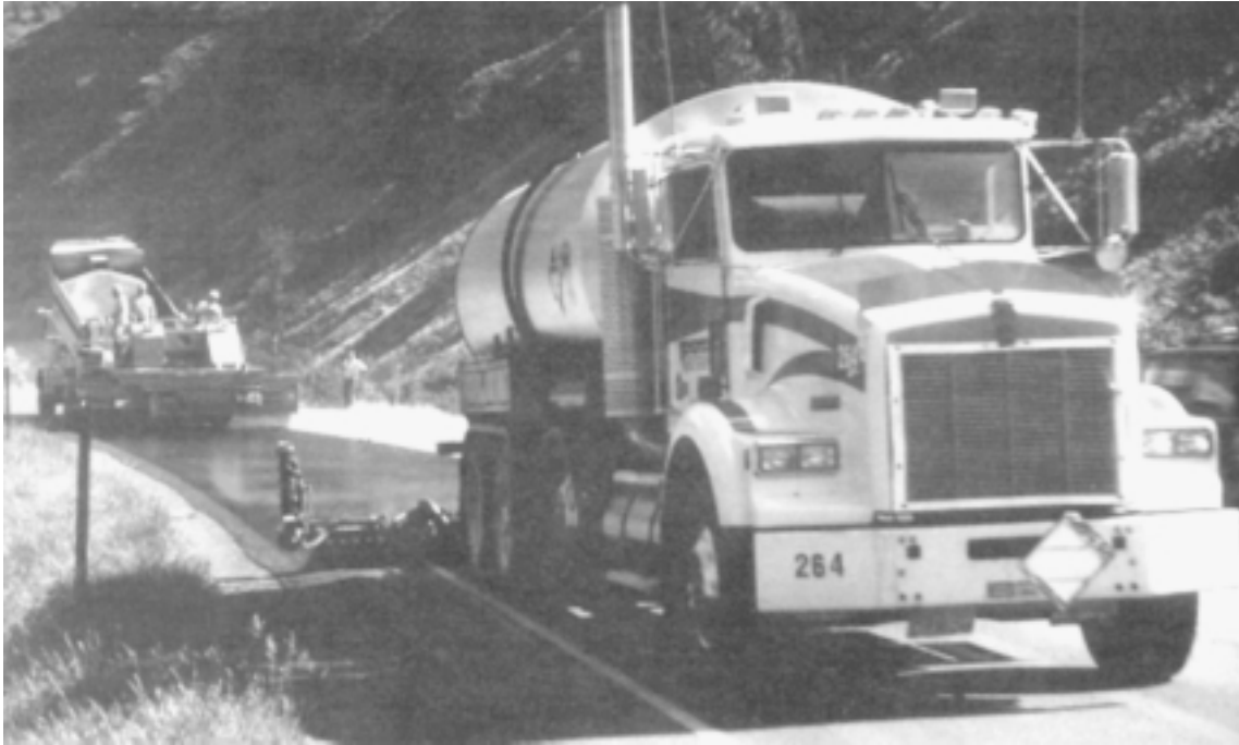
Figure 7—Chip seal treatment. (Photo courtesy of Asphalt Institute.)
