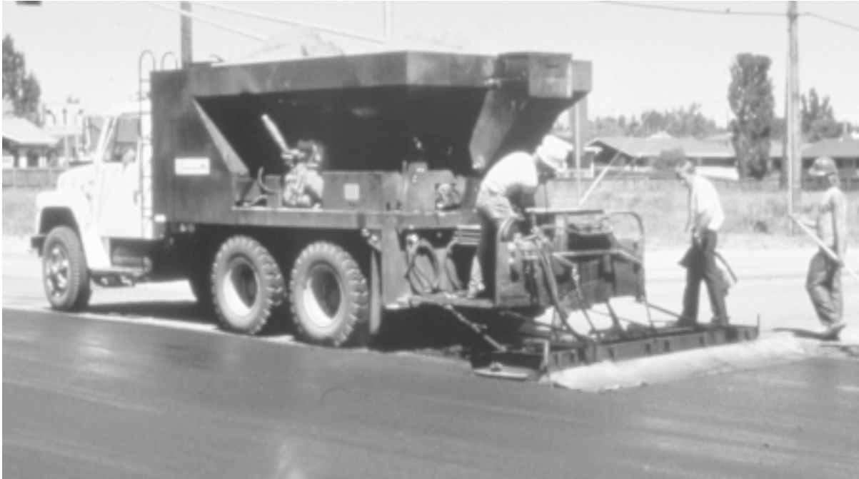
Figure 8—Slurry seal application. (Photo courtesy of Asphalt Institute.)
