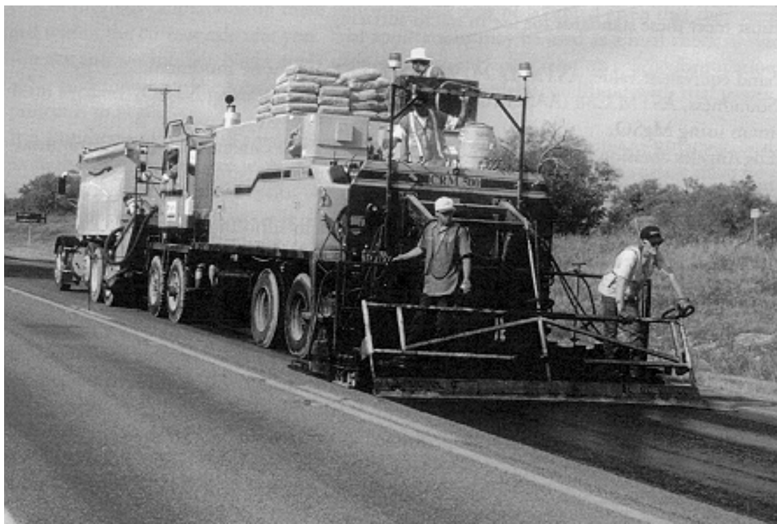
Figure 10—Microsurfacing operation. (Photo courtesy of Asphalt Institute.)
