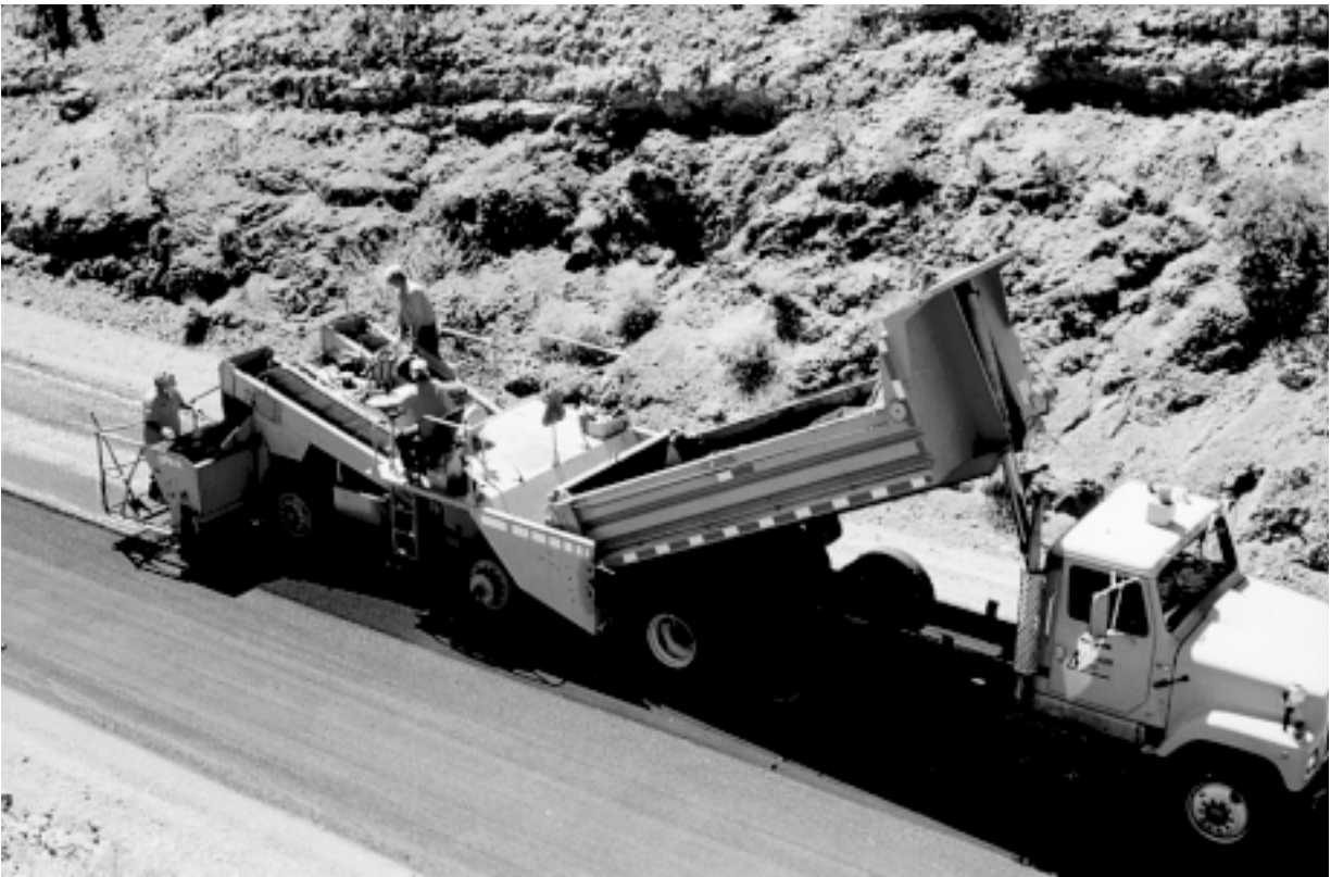
Figure 4—Sand seal. (Photo courtesy of Western Emulsion.)
