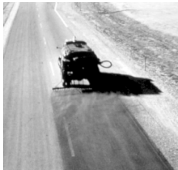
Figure 3—Fog seal. (Photo courtesy of Asphalt Institute.)
