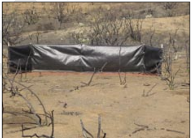
Figure 35—A recently installed silt fence.
