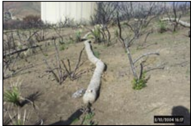
Figure 31—To ensure proper installation, work with experienced crews and inspect as the fiber rolls are installed. Improper installation negates the effectiveness of this expensive treatment.
