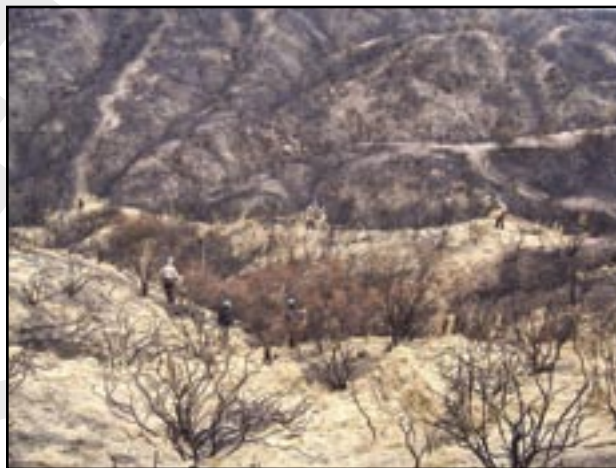
Figure 12—Crew applying straw by hand.
