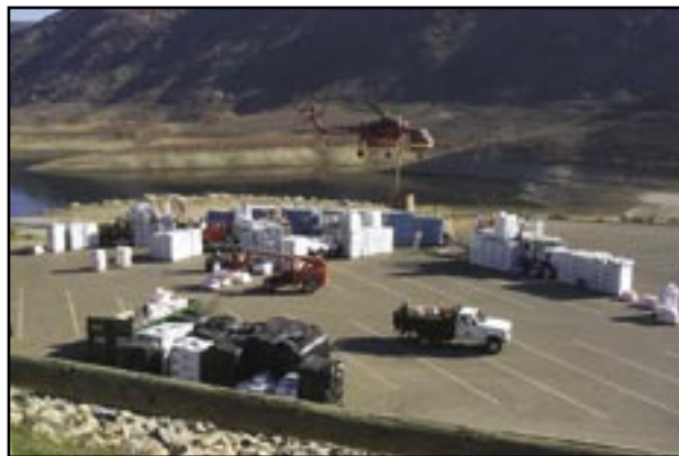
Figure 3—Aerial hydromulching requires close access to water, large staging areas, and close proximity to treatment units.
