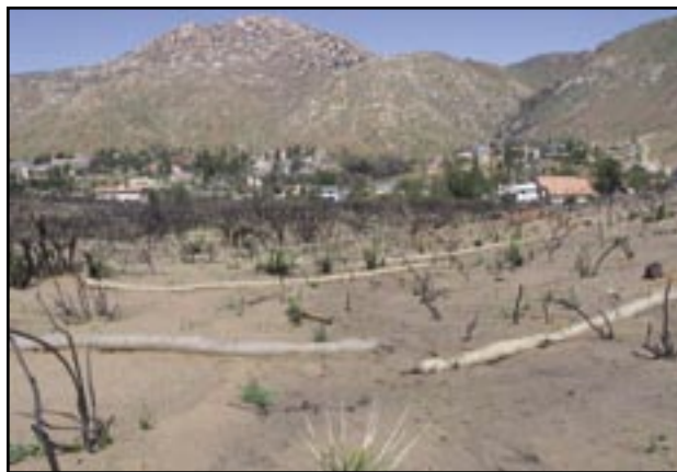
Figure 30—Fiber rolls do not reduce erosion but trap sediment on the slope. Where high values are at risk identify the emergency objective and select the treatment which best meets that objective.
