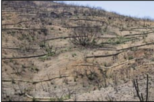
Figure 28—Fiber roll placed across the hillslope. Not all the fiber rolls are on the contour which can accelerate erosion.
