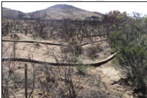
Figure 29—Avoid placing the fiber rolls in drainages.
