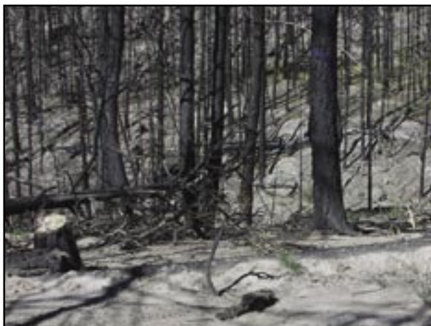
Figure 22—Contour felled LEB held in place with existing tree and stump.
