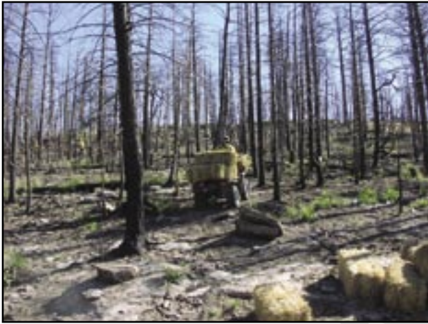
Figure 25—Area initially treated with LEBs, but secondary treatment of straw mulch is added to reduce erosion.
