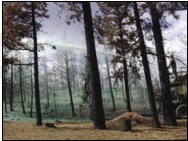
Figure 6—Ground application of hydromulch.
