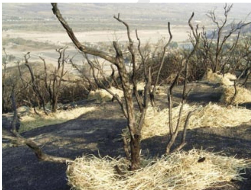
Figure 14—In windy areas straw will move offsite, leaving the soil prone to erosion.
