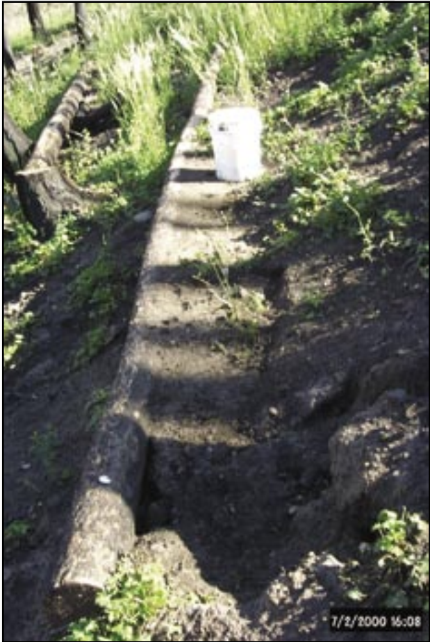
Figure 26—Contour felled LEB which has filled with sediment and then failed. Sediment trapping ability of LEBs on steep slopes is limited.
