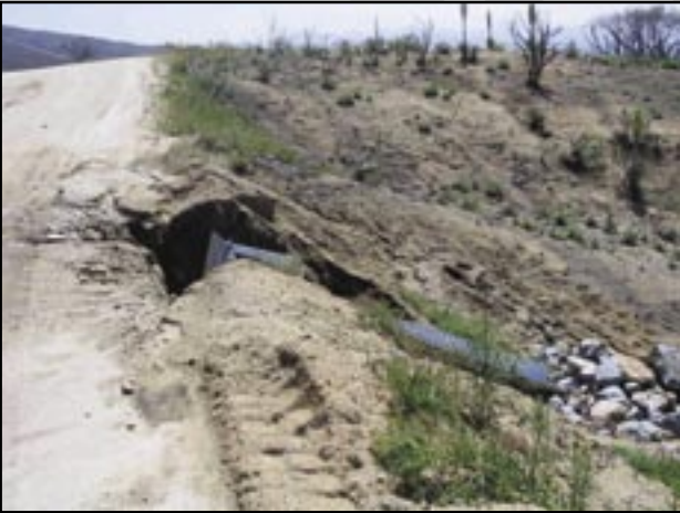
Figure 71—Failed metal roadside drain.
