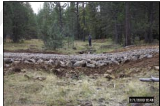
Figure 69a—Completed armored rolling dip.
