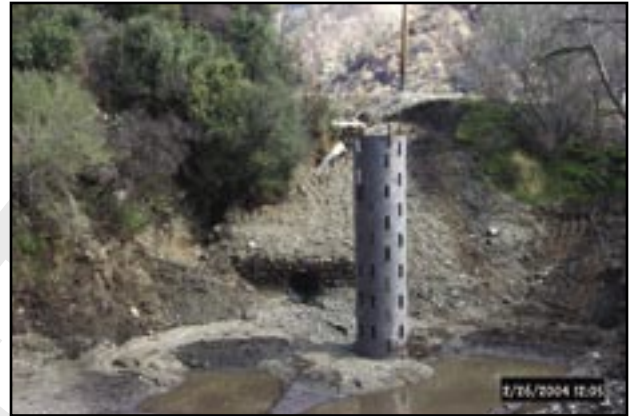
Figure 89—Riser located next to county road and receives frequent maintenance to remove material.
