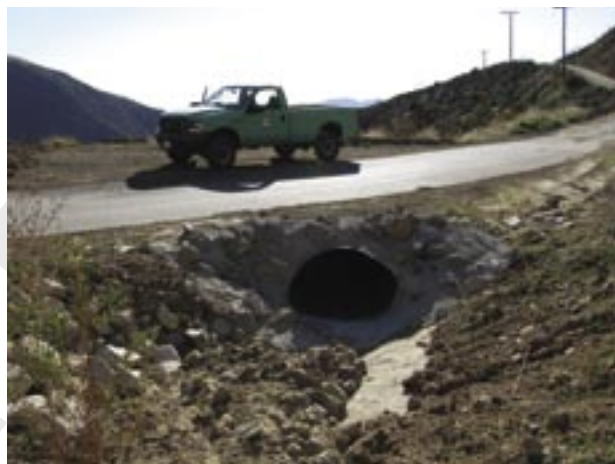
Figure 79—This larger pipe was installed to replace an undersized culvert that had failed in the past.
