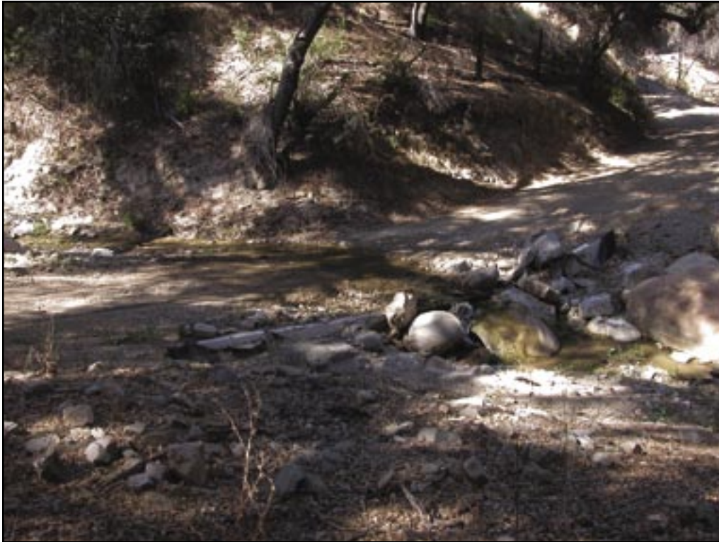
Figure 76—Low water stream crossing replaces a 24-inch culvert.
