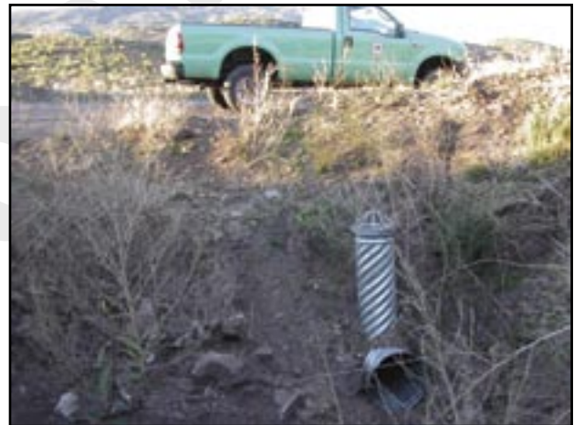
Figure 90—Small riser used to prevent plugging of culvert.
