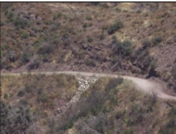
Figure 72—Rock armor used to replace failed roadside drain.
