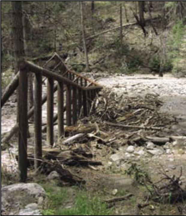
Figure 82—Debris rack effectively trapping material from plugging the culvert.
