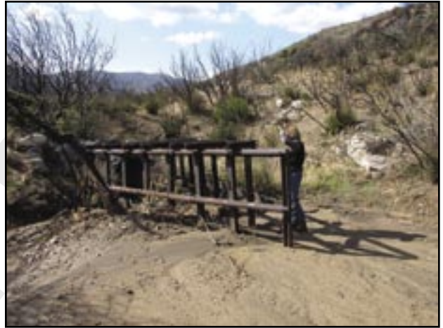
Figure 84—Debris deflector is located at inlet of culvert..
