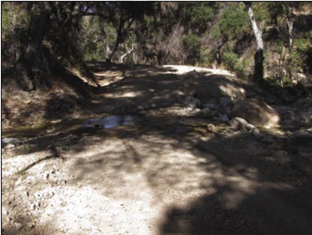
Figure 77—Ensure adequate length of the endwall and armor the outlet to prevent scouring.
