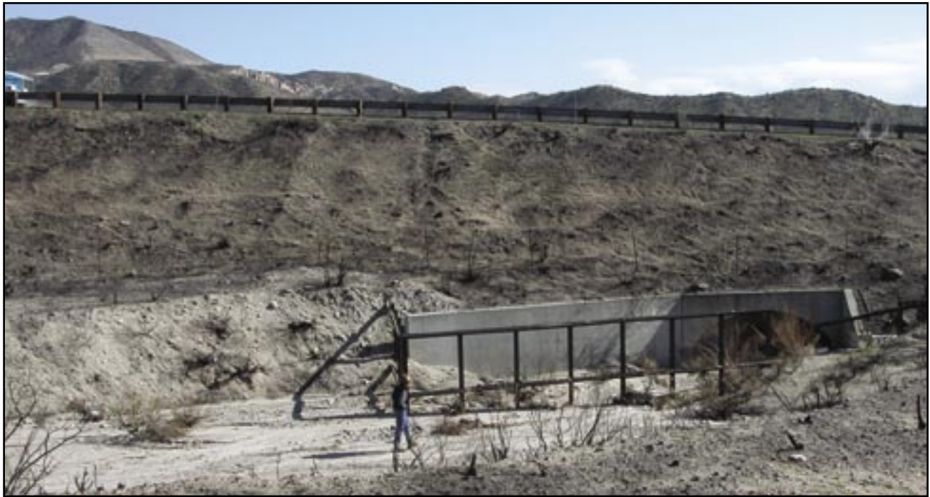
Figure 85—Large debris deflector on crossing below a major interstate.
