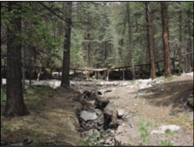
Figure 83—Debris racks must be long enough to avoid material from outflanking the structure.
