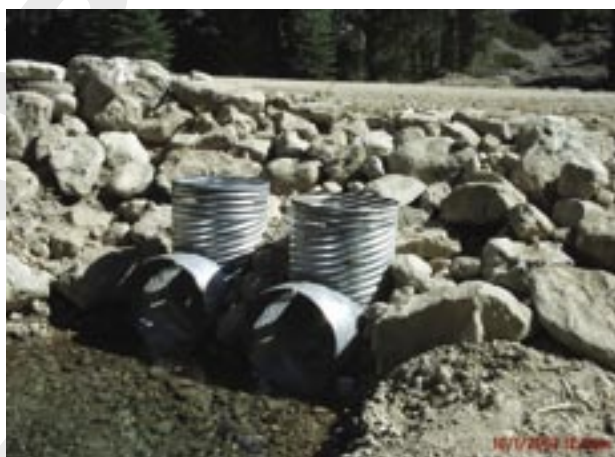
Figure 80—This culvert was modified with two culverts and risers to handle increased flows and potential woody debris.
