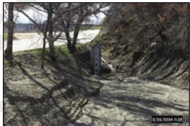
Figure 91—Riser is attached to the culvert headwall to reduce culvert plugging.
