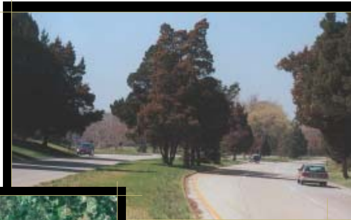
Trees and shrubs were planted in this median to visually separate the lanes of traffic and to blend the road corridor into the existing landscape. George Washington Memorial Parkway, VA
