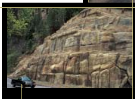
Most visitors traveling through Oak Creek Canyon would never know that this rock outcrop was sculpted concrete. Sedona–Oak Creek Canyon Scenic Road, AZ
