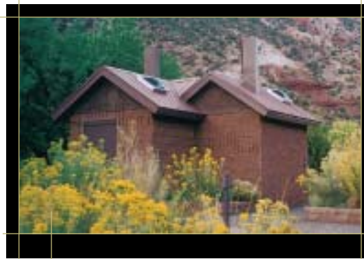
The stepped pattern and color in the hills are reflected in the color and brick pattern of this restroom. Jemez Mountain Trail, NM
