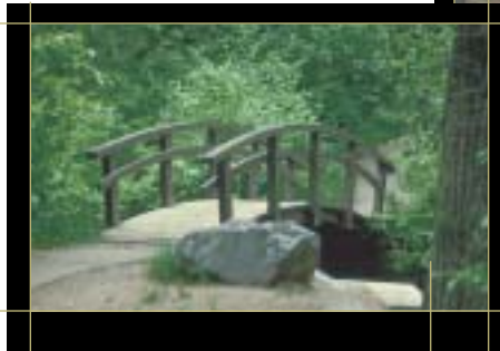
This simple arched bridge is appropriate along more developed trails with a hardened surface. The low arch makes this bridge universally accessible. Uinta National Forest, UT
