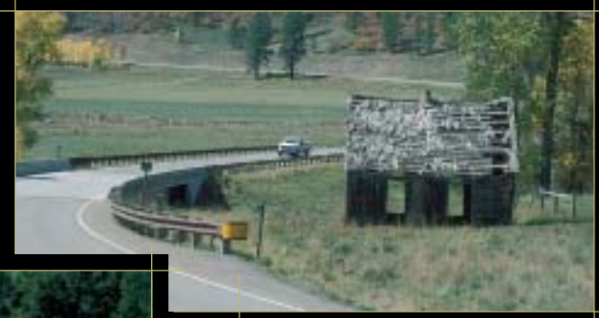
The horizontal alignment on West Delores Road curves around a historic structure to preserve it. San Juan National Forest, CO
