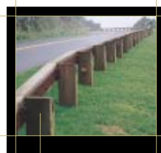
Steel-backed wooden guardrails are used to replicate the look of historic guardrails. Blue Ridge Parkway, VA
