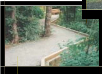
Simple timber retaining walls were used to wind this trail through the woods. Spirit Lake Memorial Highway, WA
