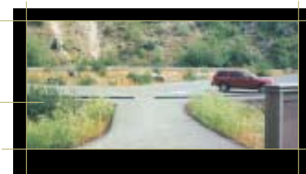
A biofiltration pond was incorporated into the design of this parking lot and planted with native plants. Spirit Lake Memorial Highway, WA
