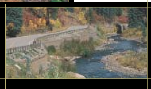
This welded-wire retaining wall along the West Delores Road was chosen because the color of the stone blends into the environment, and it was less expensive than a concrete wall. San Juan National Forest, CO
