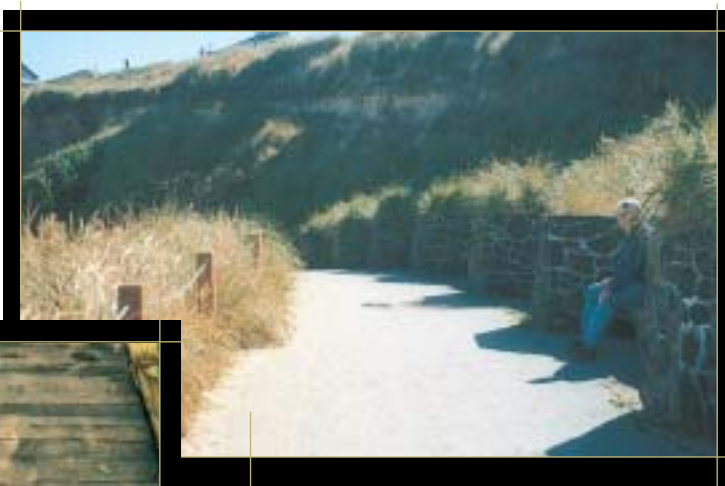
The retaining wall along this trail incorporates benches set back from the trail that are visually separated from each other, making them more private. Newport, OR
