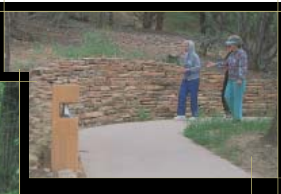
This native dry-laid stone retaining wall with its irregular height makes an attractive transition from the natural landscape to the paved trail with lighting. Ridgway State Park, CO
