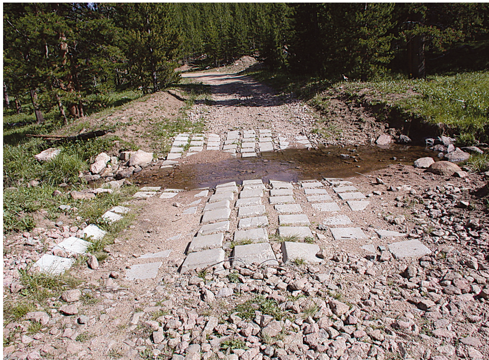
Figure 5.6—Cable concrete block ford, Bighorn National Forest, Wyoming. Note that mat should extend higher to protect the crossing adequately.
