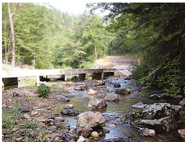
Figure 5.14—Long Creek embedded concrete box high-VAR ford constructed in 2005, Ouachita National Forest, Arkansas.
