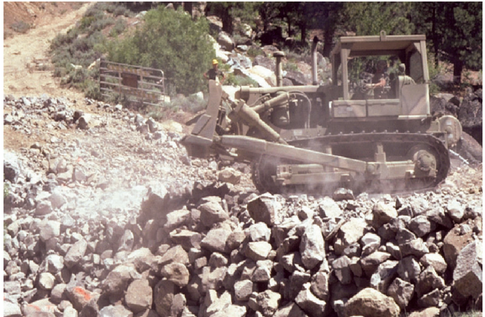
Figure 5.9—Dooley rockfill ford under construction, Plumas National Forest, California.
