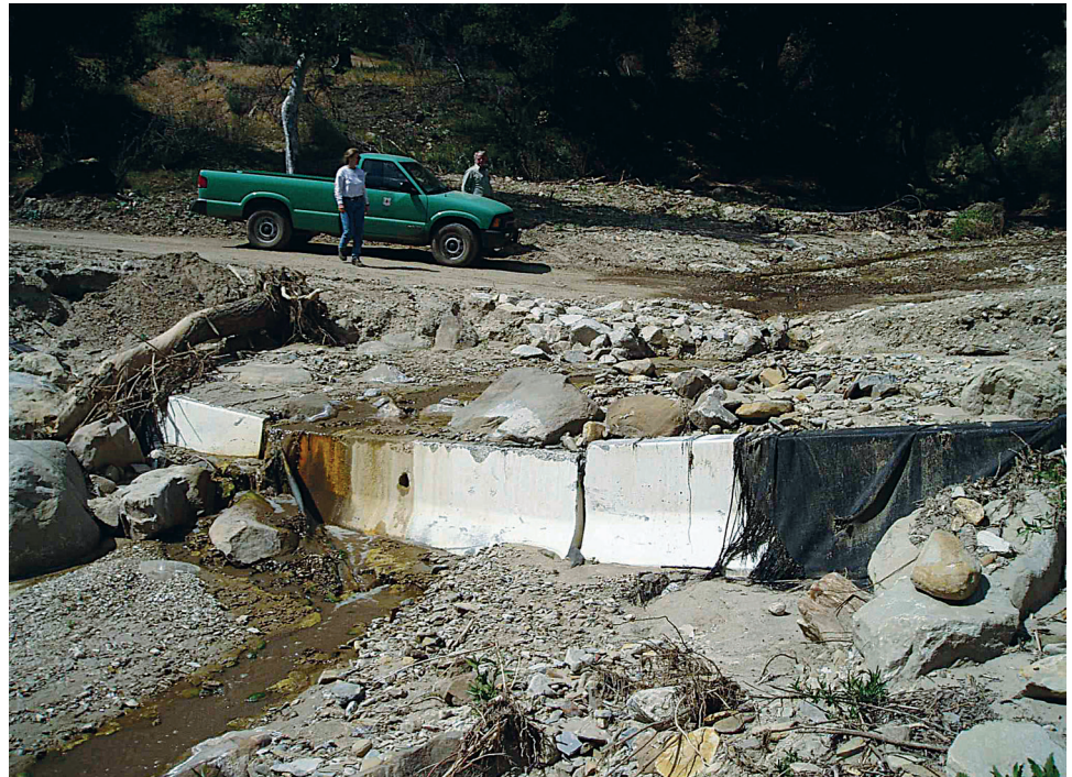
Figure 5.12—Jersey barriers used for a temporary ford after the Ojai wildfire in 2004, Los Padres National Forest, California.
