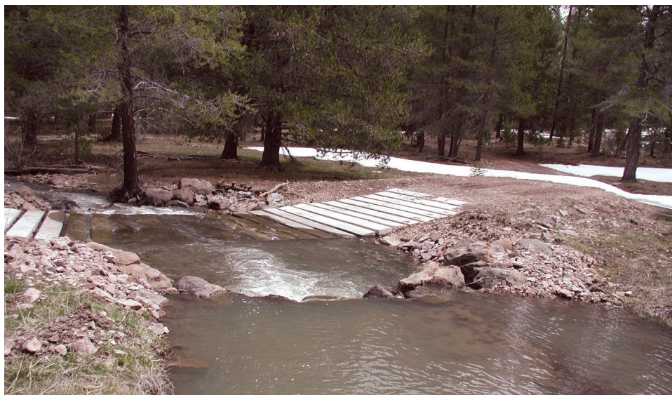
Figure 5.4—The Thomas Creek 198 ford, Fremont National Forest. A slot in the concrete slab between the planks provides low-flow passage for trout.
