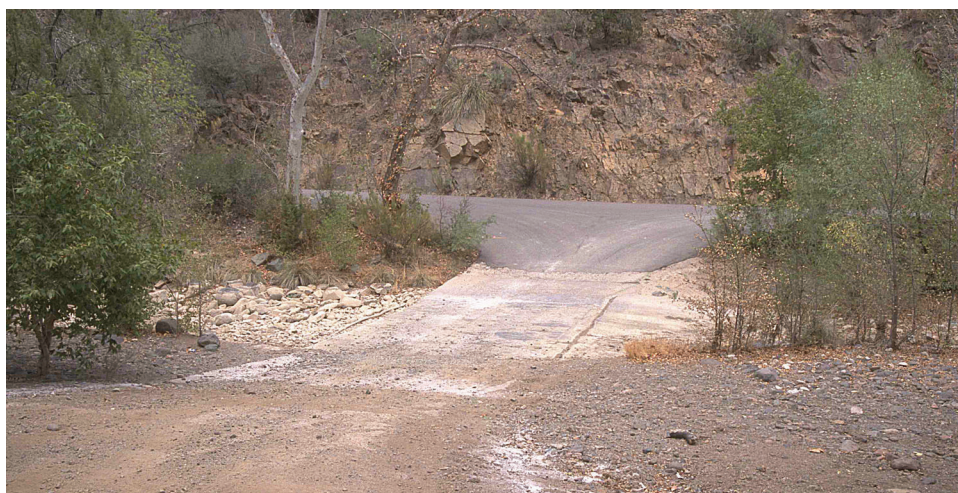
Figure 5.3—Old concrete slab ford with grout apron, Ashdale Administrative Site, Tonto National Forest. (case study 8)
