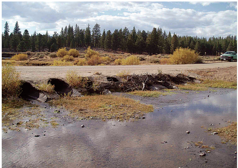
Figure 5.13b—Murdock ford, looking downstream at inlets partially plugged with woody debris after a high flow.
