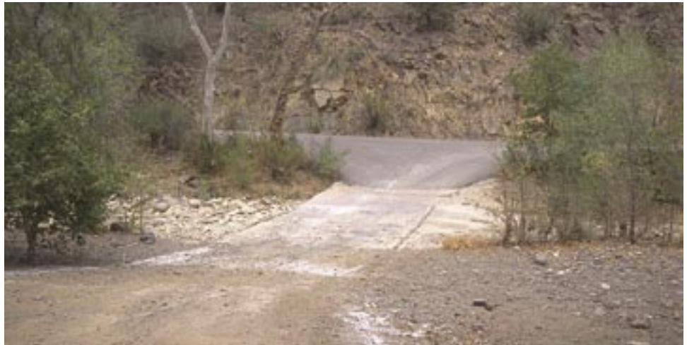
Figure 5.3—Old concrete slab ford with grout apron, Ashdale Administrative Site, Tonto National Forest. (case study 8)
