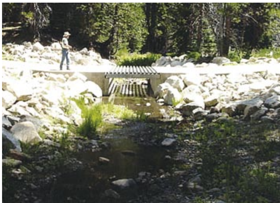
Figure A80. One of several grating-top box culvert fords on tributaries of the North Fork Consumnes River.
