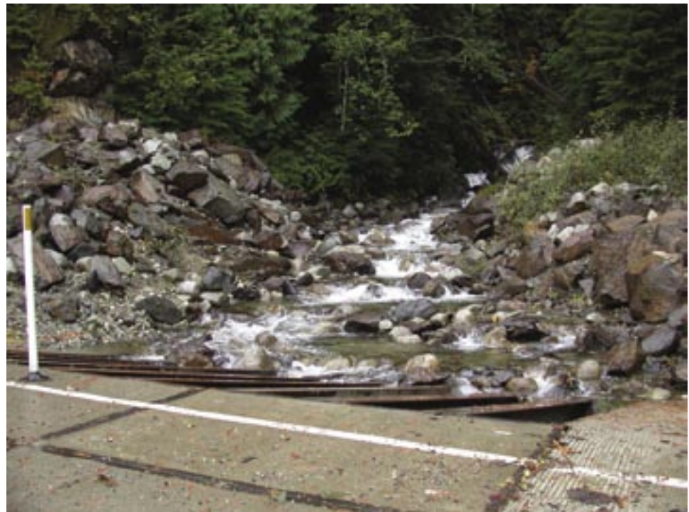
Figure A109. Sibley Creek currently approaches the inlet at a slight angle.
