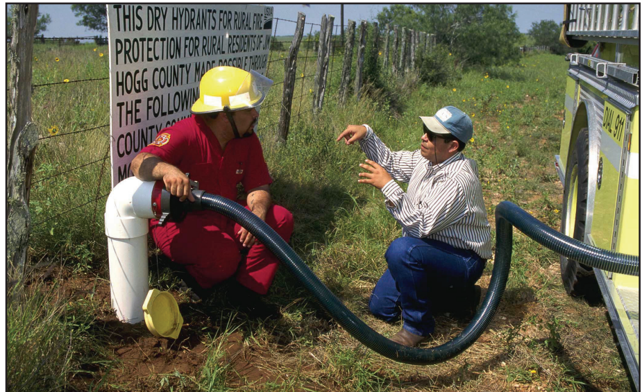
Figure 19—Dry hydrant.
