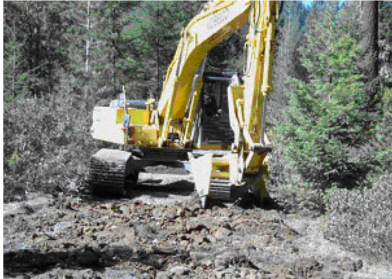
Figure 6a. Road obliteration using the SEB.
