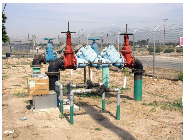
Figure 55—Backflow prevention valves.
