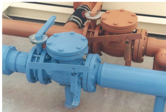
Figure 47—Check valves.
