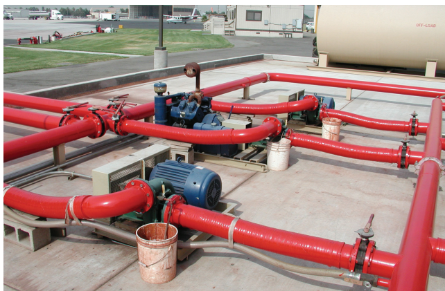
Figure 48—Electric- and gasoline-powered retardant pumps with vibration isolating flexible hose (San Bernardino, CA).
