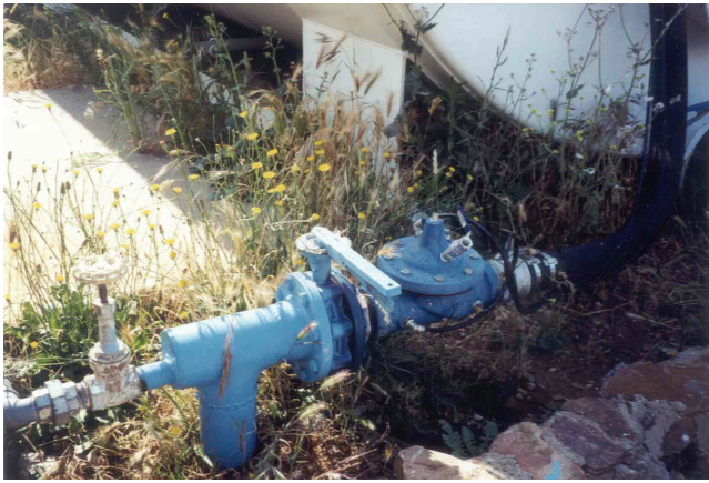
Figure 56—Automatic water valve.
