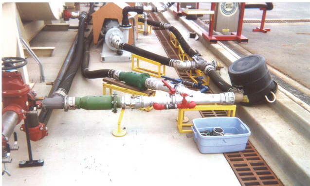
Figure 43—Liquid product delivery system with wye blender (JEFFCO, CO).
