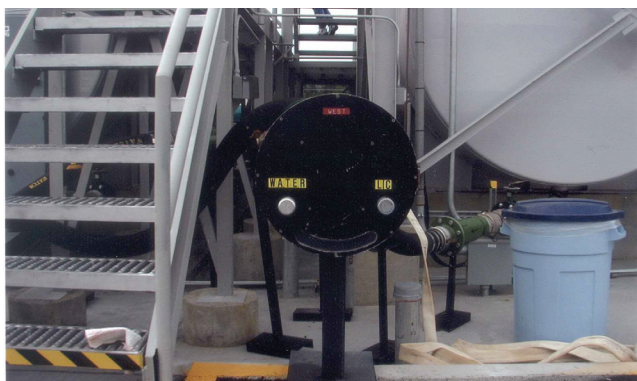
Figure 46—Inline proportioner, Vari-blender (McCall, ID).
