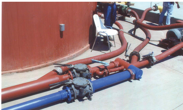
Figure 44—Inline proportioner, orifice blender (Redmond, OR).
