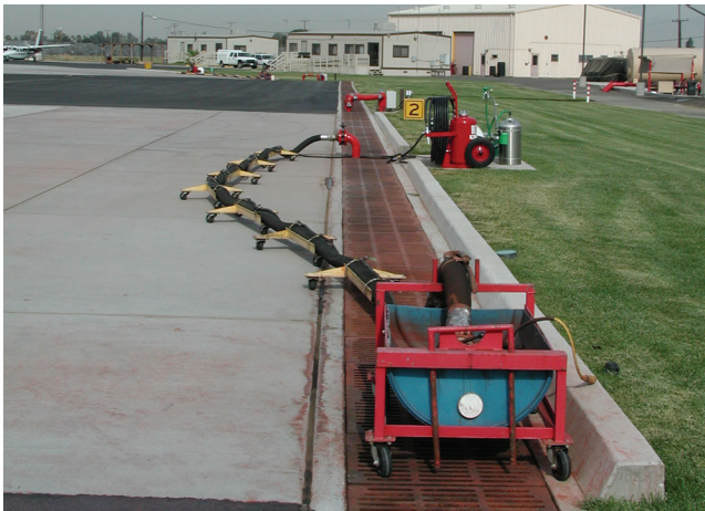
Figure 30—Loading pad wash down water collection trench with grating (San Bernardino, CA).
