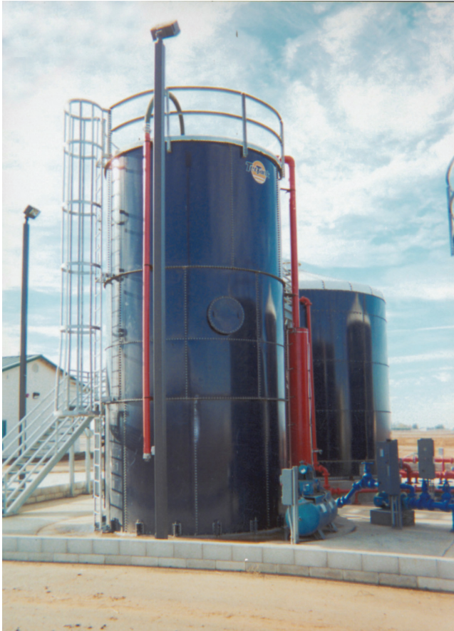
Figure 17—Dry powder retardant storage silo (Porterville, CA).
