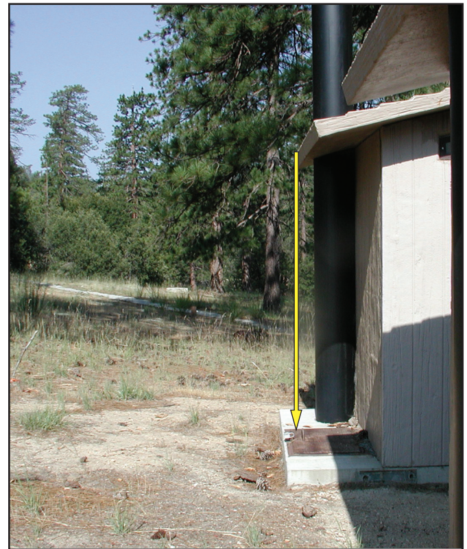
Figure 1—The roof dripline is directly over the manhole lid in the single vault CXT toilet building.
