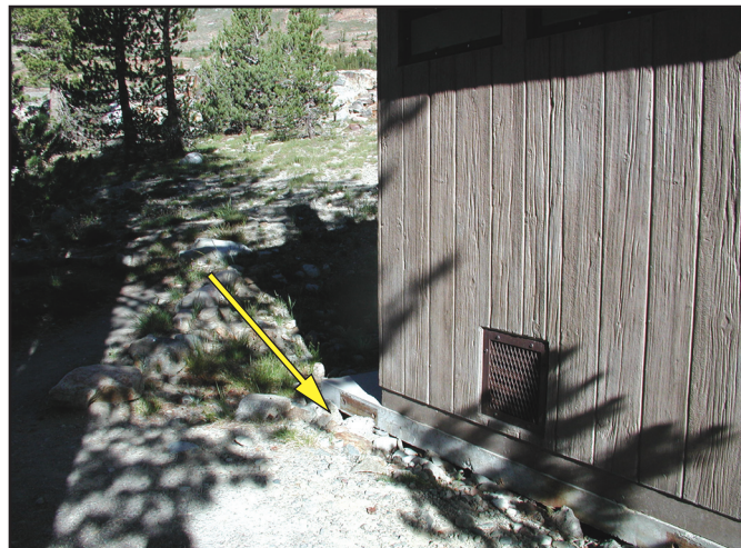
Figure 6—This vault is below finished grade. The mastic between the building slab and vault is damaged. The vault fills with water every spring.
