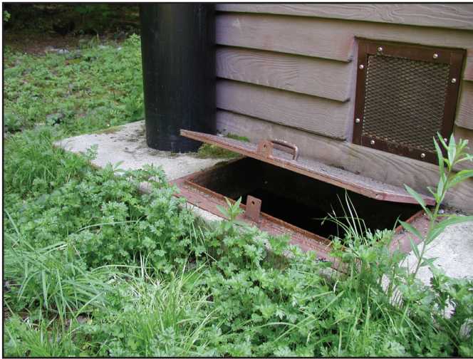
Figure 8—Retrofit “shoebox” lid stops water from entering the vault by going under the lid.
