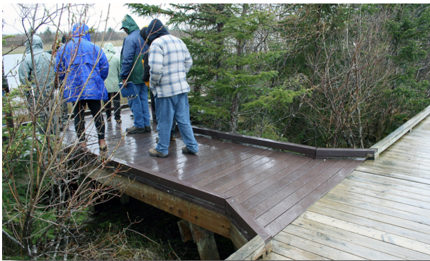
Figure 6—Alaska boardwalk shows a combination of plastic wood with natural wood.
