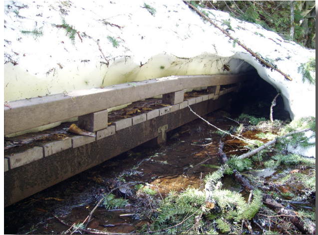
Figure A.4—The puncheon in May 2008 after a winter of very heavy snow loads. After the snow melted and some summer heat, it bounced back to normal (or so close to normal it's not noticeable).
