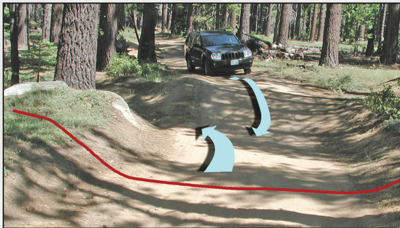
Figure 3.11—Broad-based dip breaks up contributing area and reduces maintenance frequency.
