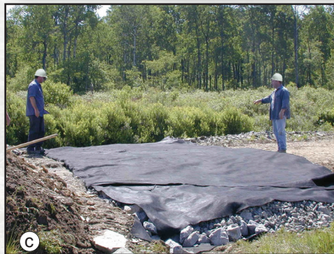
Figures 2.16a through 2.16d—French mattress construction sequence.
