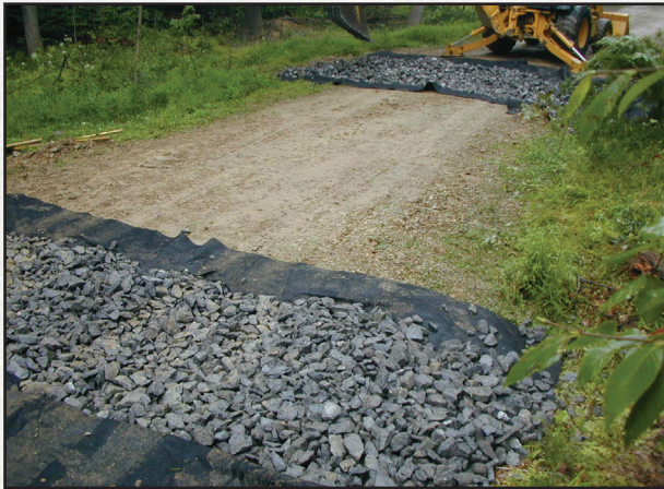
Figure 2.15a—Small mattresses installed to drain several springs and seep.
