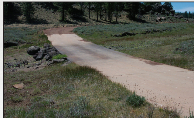
Figure 6.5—Concrete ford crossing.
