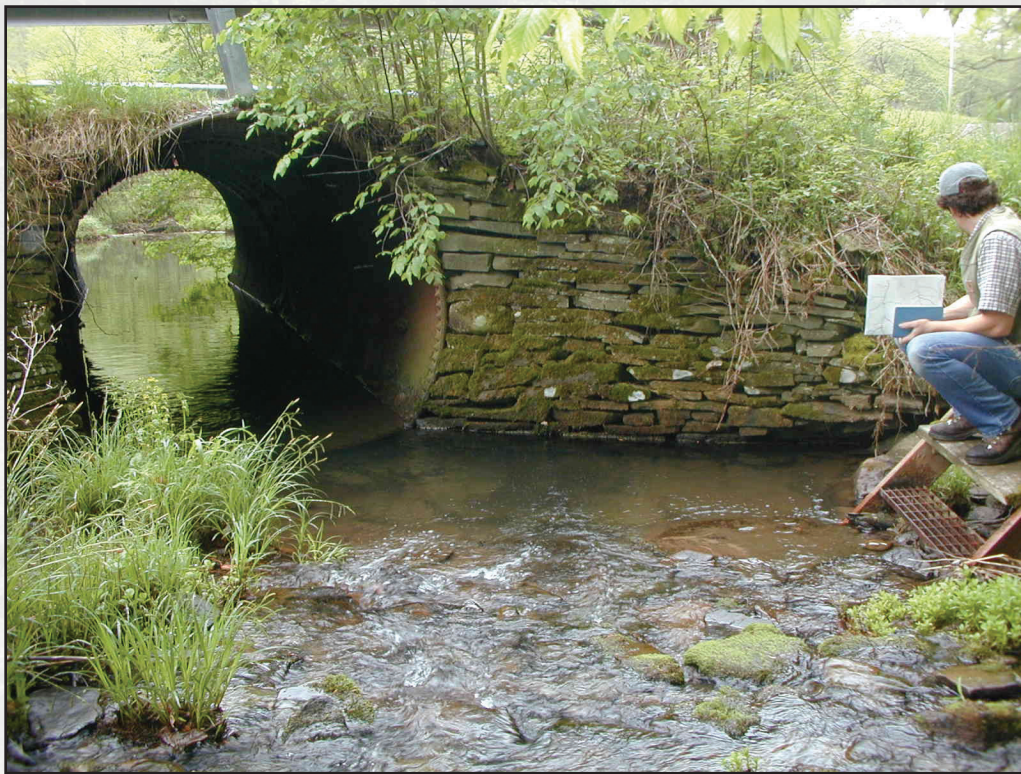
Figure 5.13—A properly constructed natural stone headwall can last for decades.
