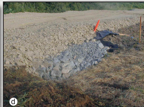
Figures 2.16a through 2.16d—French mattress construction sequence.
