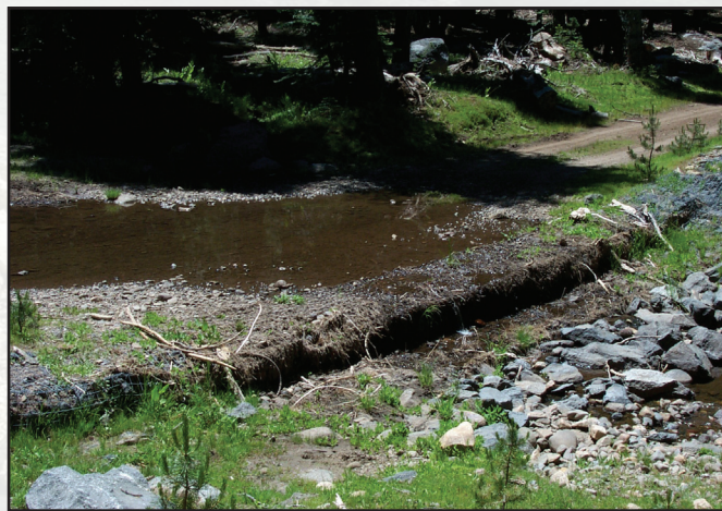
Figure 6.8—Gabion ford crossing.
