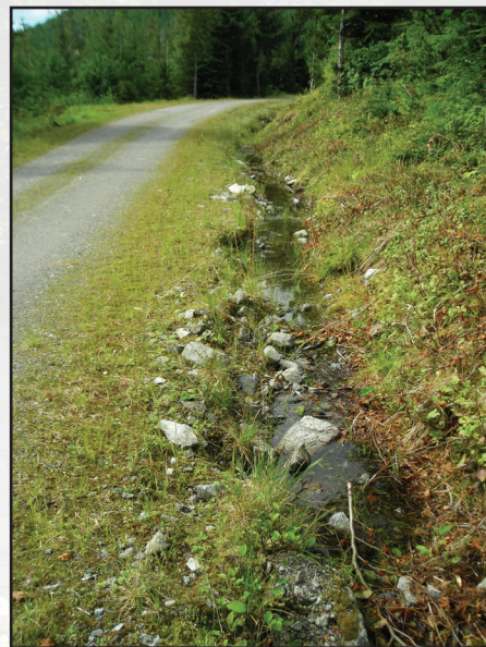
Figure 2.4—Road ditch with standing water.
