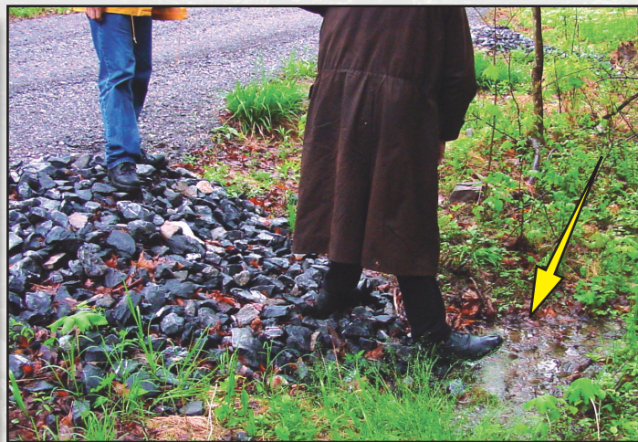
Figure 2.14—This is the same mattress outlet after completion. Notice the water flowing out of the mattress below the road.
