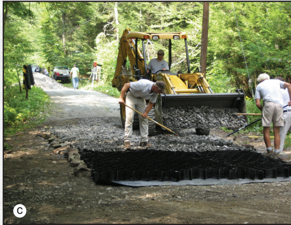
Figures 6.4a through 6.4d—Construction sequence for high-water-bypass.
