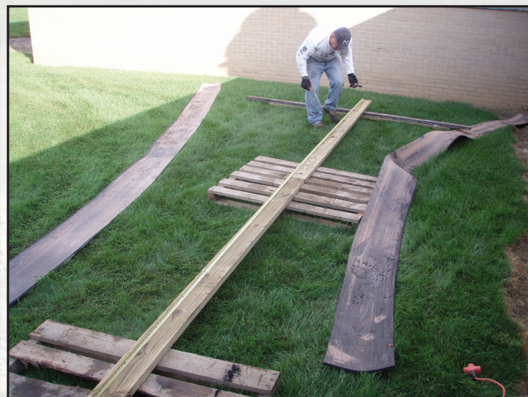
Figure 3.17—Construction of a 24-foot-length diversion. Note that the belt has been cut in half lengthwise. A 4-foot board on top of the belt spans the lumber joint of two 12-foot boards.
