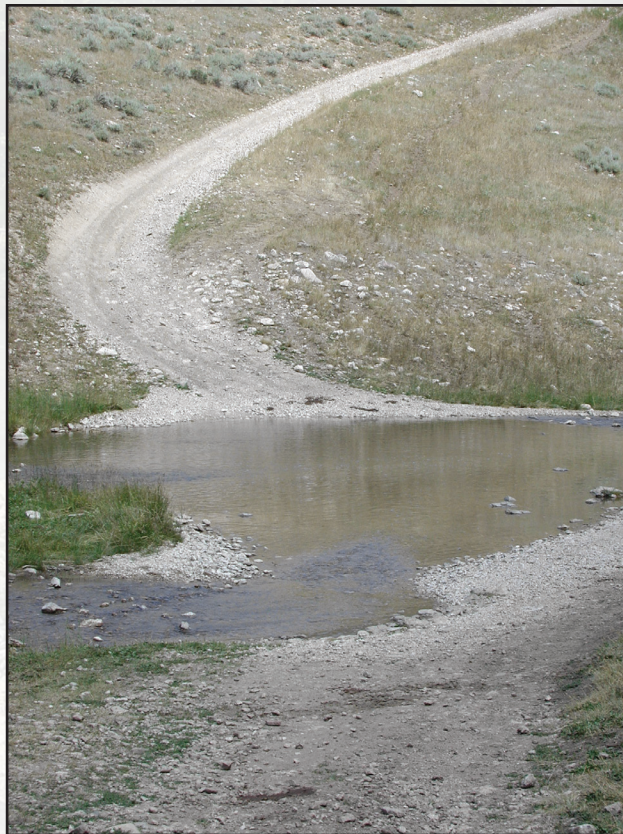
Figure 6.3—This direct road-stream connection causes deteriorated water quality and adverse impacts to aquatic species, animals, and humans.
