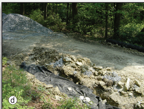
Figures 2.8a through 2.8d—French drain construction sequence.
