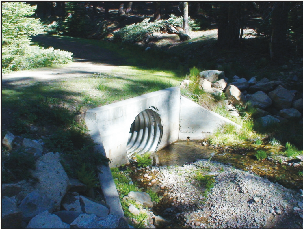
Figure 5.14—Headwall with wingwalls.
