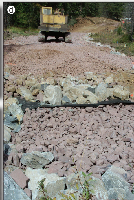
Figures 2.22a through 2.22d—Permeable fill construction sequence.
