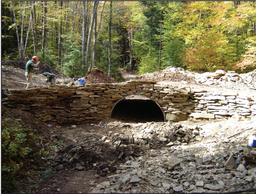
Figure 6.12—A bottomless arch pipe has just been installed over a currently dry stream channel.
