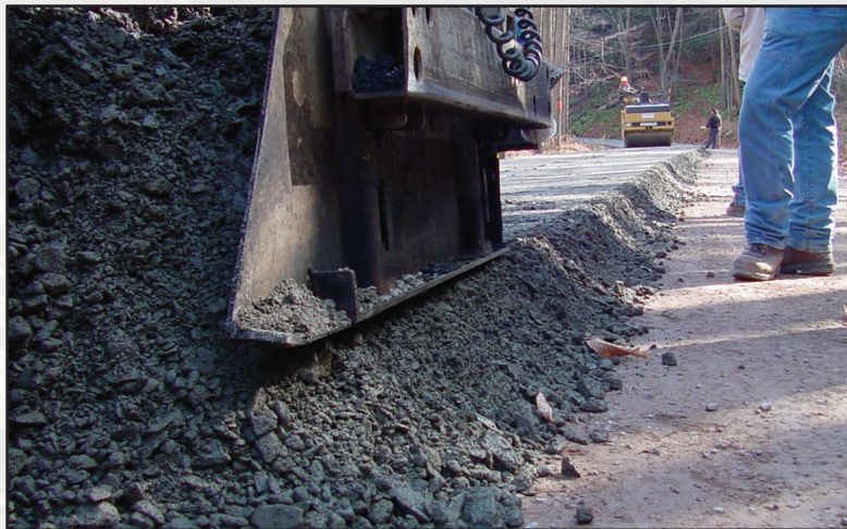
Figure 8.5—A well-graded aggregate is being placed through a paver at a noncompacted depth of 8 inches, and compacted to 6 inches. Notice the roller in the background for compaction.
