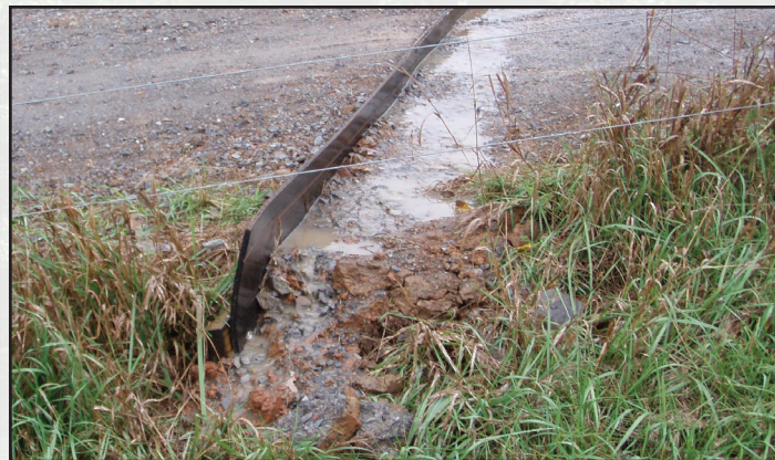
Figure 3.15—A completed diversion directs surface drainage off the roadway and into a field.
