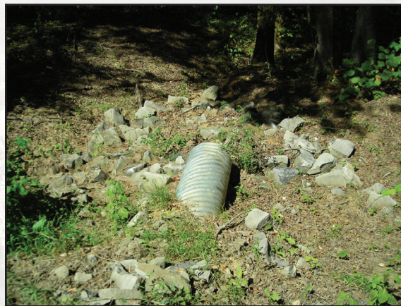
Figure 5.3—Culvert outlet is well armoured.
