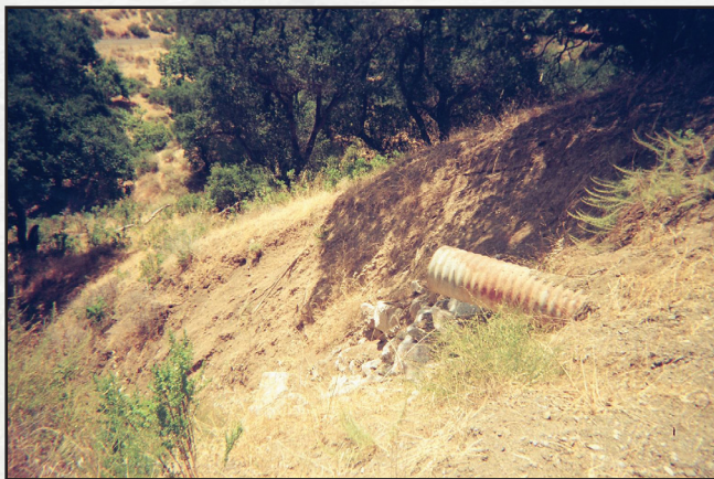
Figure 5.2—Shotgun culverts causes accelerated erosion.
