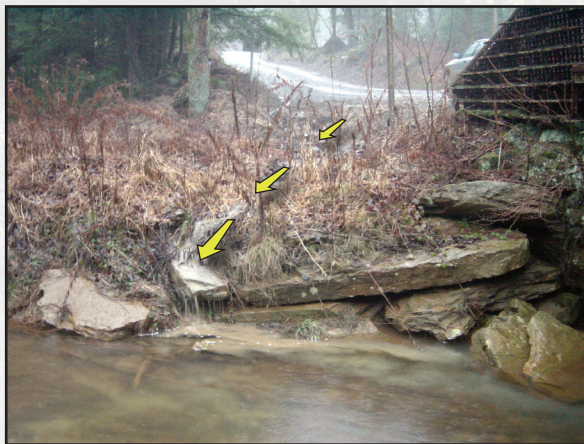
Figure 4.20—Traditional urban stormwater approaches collect and convey ditches directly to streams, as pictured above. Modern rural stormwater management should disconnect the road and stream by avoiding concentrated discharges to streams and encourage drainage dispersal.
