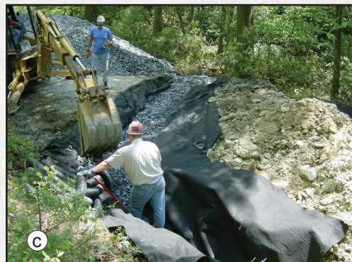
Figures 2.8a through 2.8d—French drain construction sequence.
