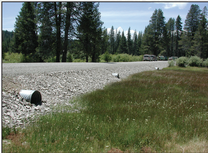
Figure 2.20—Permeable fill with culverts.
