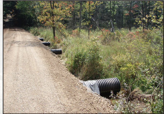
Figure 2.19—Permeable fill with culverts spreads surface flows.
