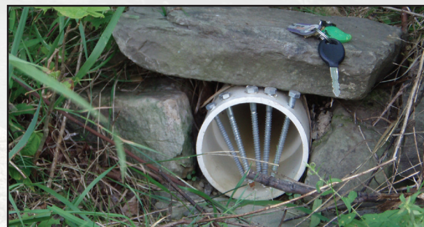
Figure 2.10—This homemade guard will prevent animals from entering the underdrain outlet.
