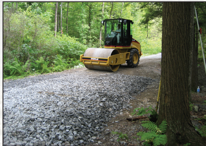
Figure 2.25—Roller compacts each of lift aggregate.
