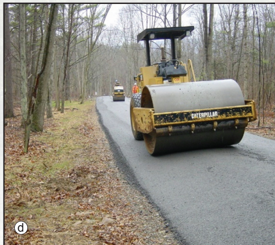
Figures 4.13a through 4.13d—Raising the road profile construction sequence.
