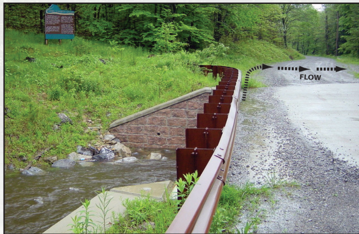
Figure 4.22b—After: Material has been added and the ditch has been reprofiled to drain away from the stream through a new cross pipe and into the woods.
