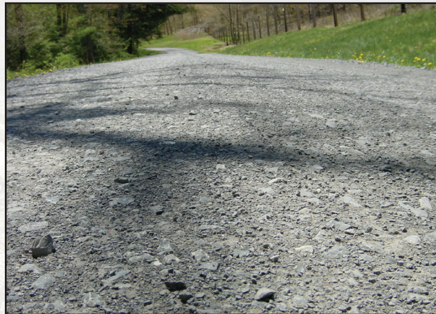
Figure 8.3—3-year-old dense packed surface aggregate after 40,000 vehicles.
