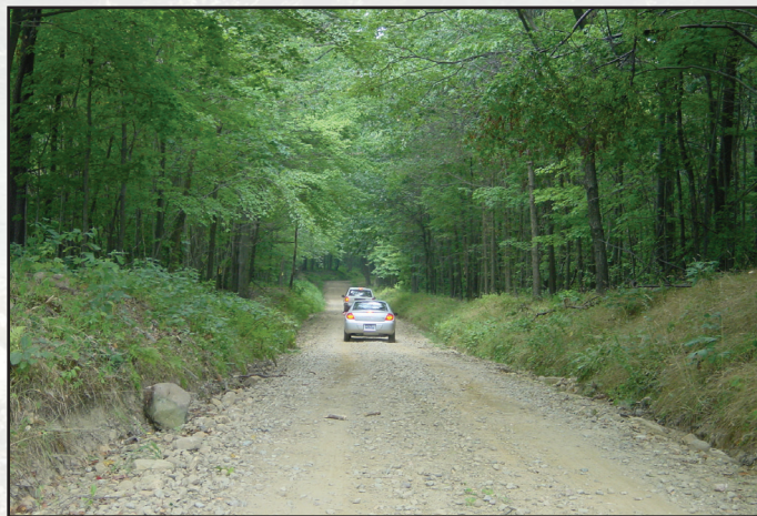
Figure 4.7—Example of an entrenched roadway.
