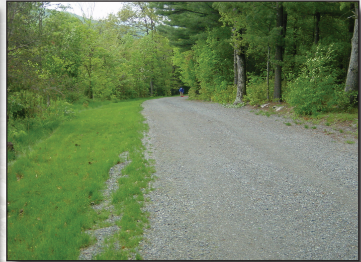
3.4b—Outsloped roads eliminates ditches.
