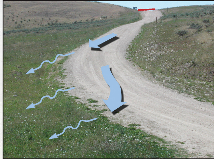
Figure 3.4a—Outsloped road disperses flow.
