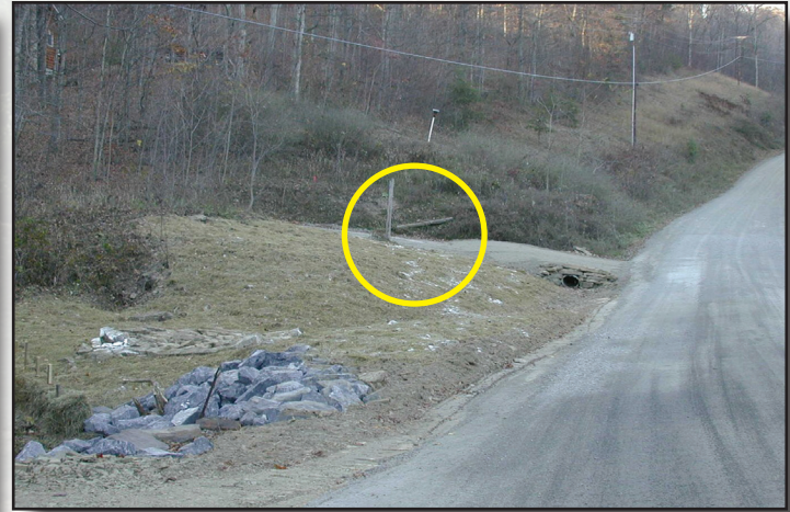
Figure 7.14—The broad-based-dip on this driveway provides a good transition and keeps water off the public road.
