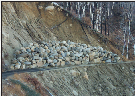
Figure 7.6—Crib wall stabilizes this steep cutslope ensuring appropriate road width and drainage function.
