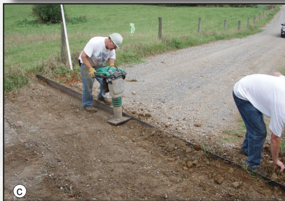
Figures 3.18a through 3.18d—Belt diversion construction sequence.
