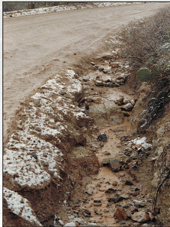
Figure 4.6—Eroded ditches are a common problem.
