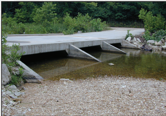
Figure 6.7—Vented ford or low-water bridge.
