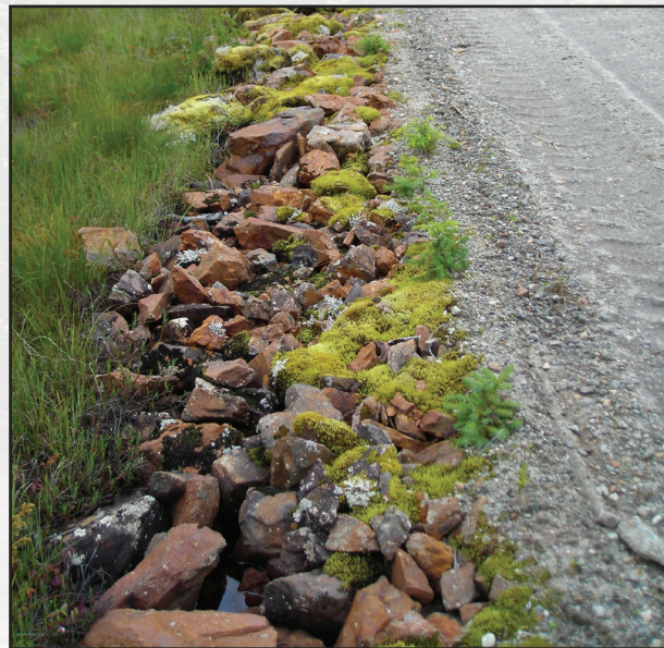
Figure 2.21—Permeable fill without culverts.
