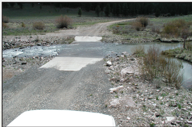
Figure 6.6— Low-water crossing.
