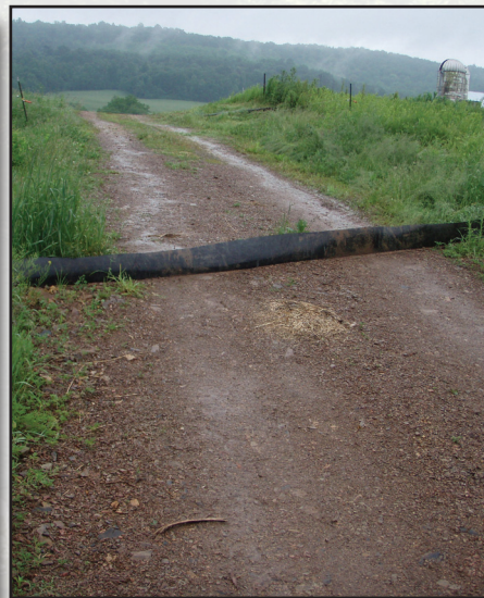
Figure 3.13—Conveyor-belt diversion on a farm lane (road).
