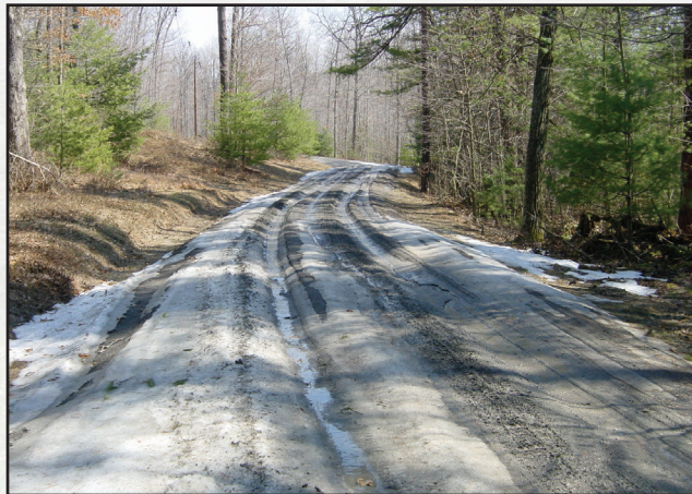
Figure 8.2—Rutting due to excess clay content.
