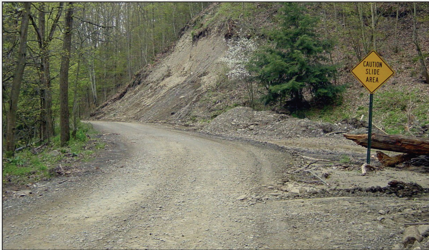
Figure 7.1—Unvegetated cutslopes are a source of sediment.
