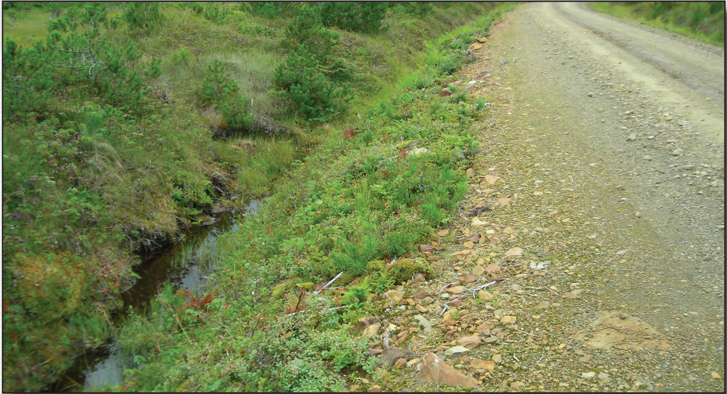
Figure 2.1—Permeable fill provides for subsurface flows.
