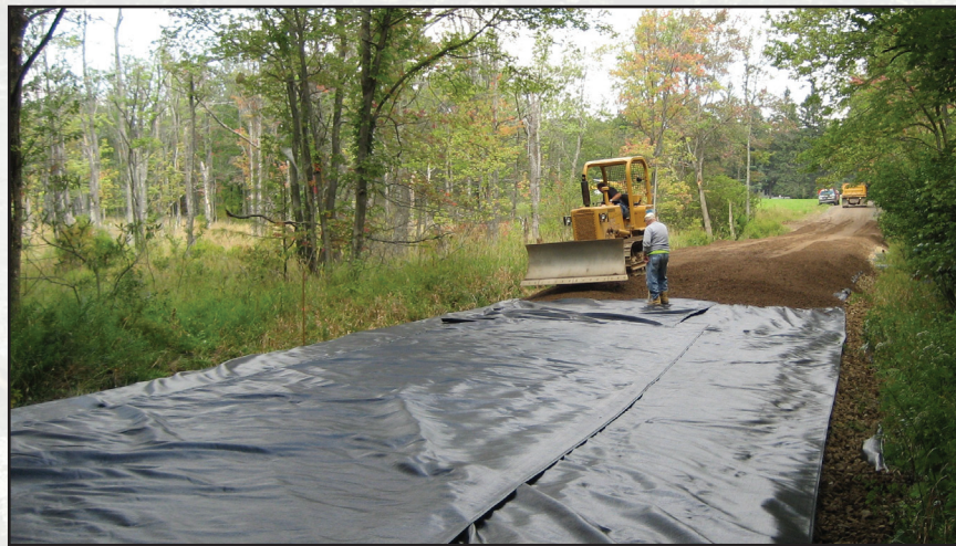
Figure 2.23—Geotextile fabric provides support for permeable fill.
