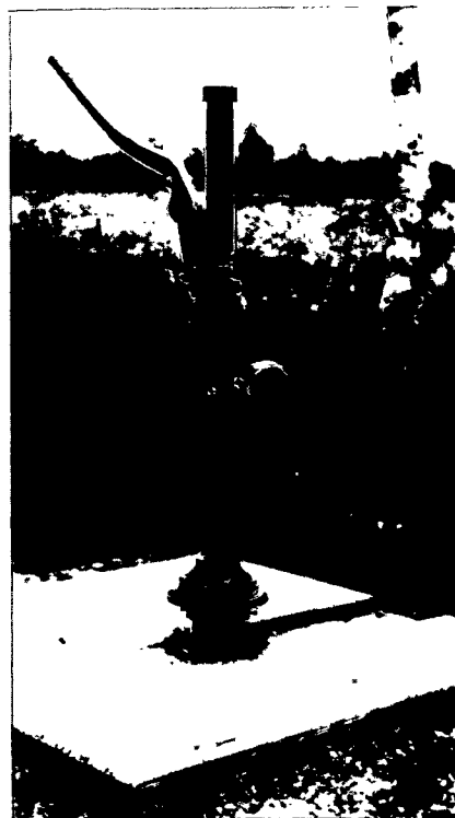
Figure 2.—Field installation of hand pump with shroud.
