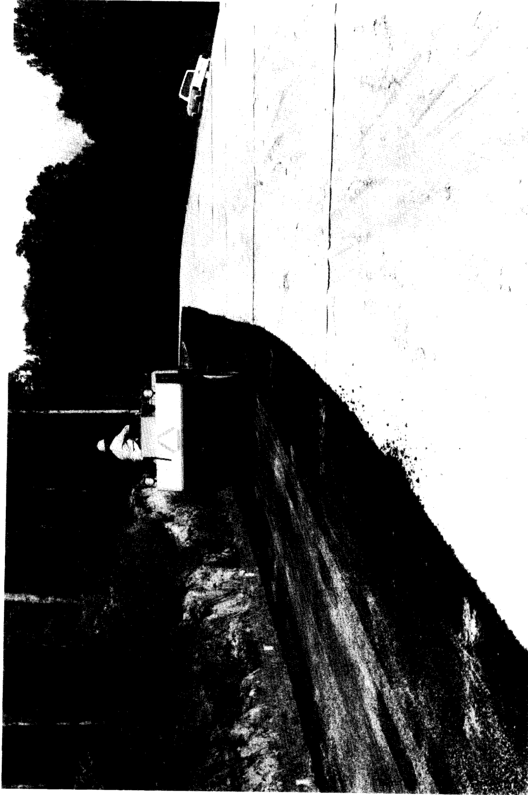
Photo 6. Compaction of the asphalt mix with a rubber-tired roller
