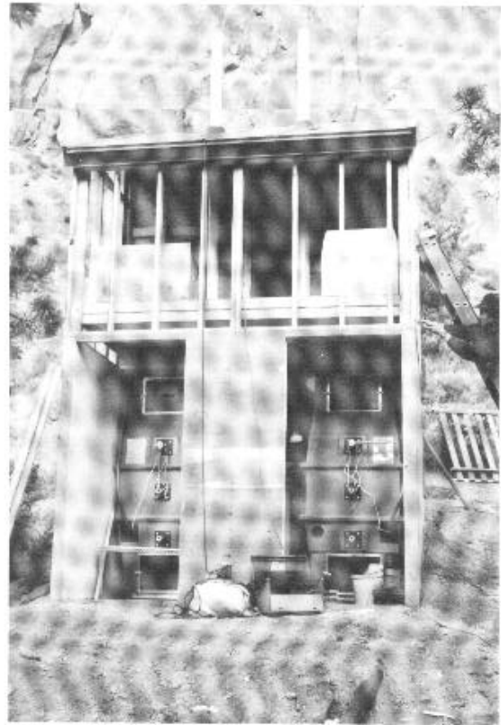
Figure 29. Smith Rock State Park, construction photo. Two Phoenix composting tanks, with two toilets, photovoltaic electrical system, compost pasteurizer, liquid evaporator, and an active solar collector built into south roof. Rainwater catchment system collects fresh water from the roof.
