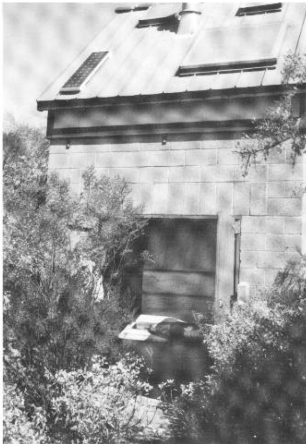
Figure 12. Organ Pipe National Monument. The double doors on this daylight basement open to allow room to maintain the compost pile. The lower service road provides access to pump the excess liquid holding tank.
