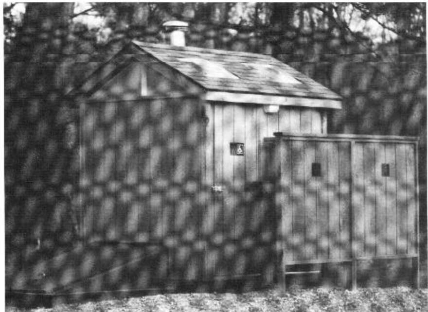
Figure 32. Alabama River Lakes, U.S. Army Corps of Engineers. Bilco doors into basement and stair access avoid a confined space area. Building from Clivus®.
