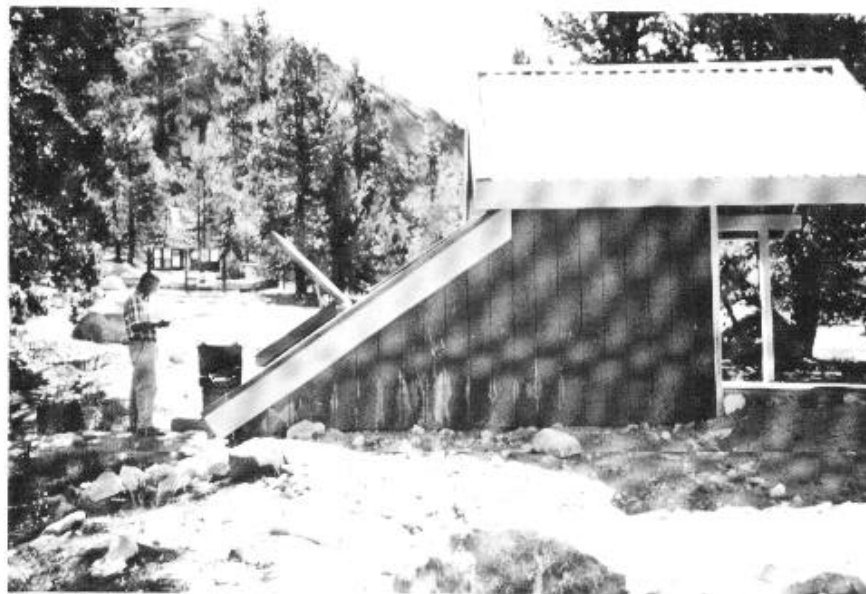
Figure 3. The hatch access to this basement results in a restricted entry. Basements with restricted entry are confined spaces and must be included on the confined space inventory. These spaces must be evaluated for potential hazards in accordance with 29 CFR 1919.146.
