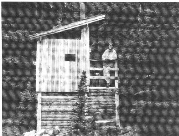
Figure 8. Yoho National Park, Canada. Recirculating solar heated air and fully insulated foundation keep the biomass warm enough to decompose at this high altitude northern location. The rustic look of cedar slab siding fits in this remote location.
