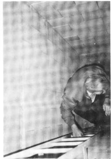
Figure 5. Ladders create restricted access resulting in confined space entry conditions.
