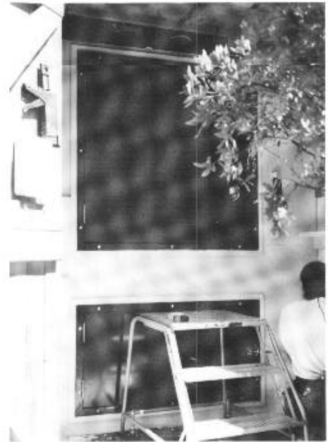
Figure 44. Yosemite National Park Site-built Composting Toilet, basement. This site-built composting toilet has large access doors for maintenance.
