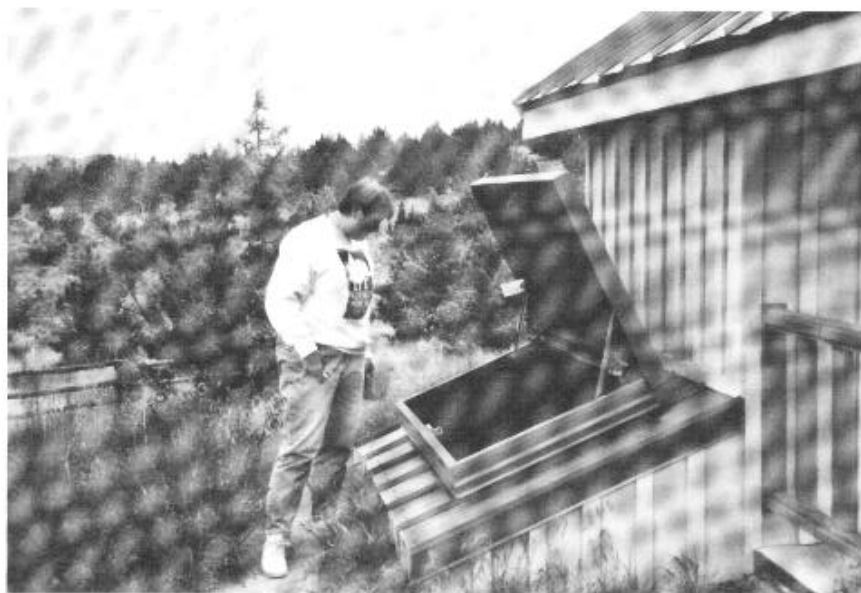
Figure 7. This basement is a "deep, dark, disgusting pit." This basement with hatch and ladder access is a confined space.
