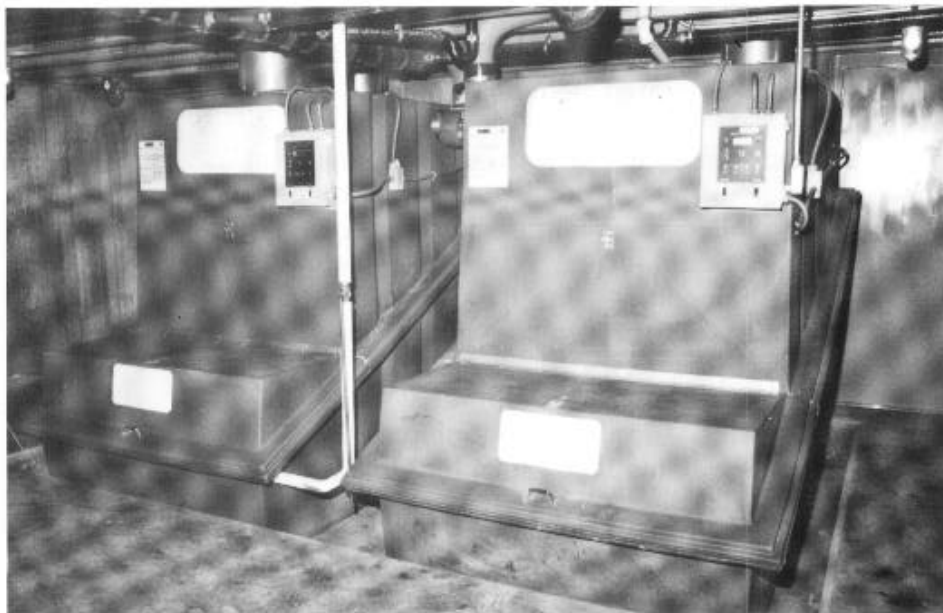
Figure 31. Clivus® Tanks, M35, installed.
