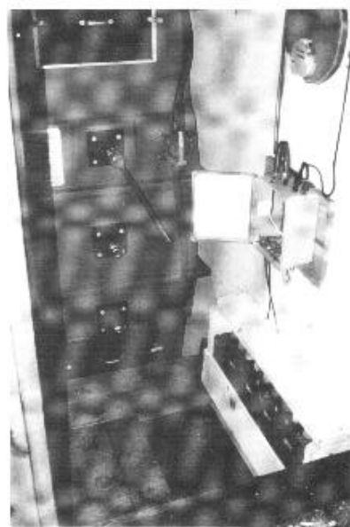
Figure 18. Flooded nicad battery bank and controls in a daylight basement. Most locations need batteries to run the forced ventilation 24 hours a day. This installation is by ACS.
