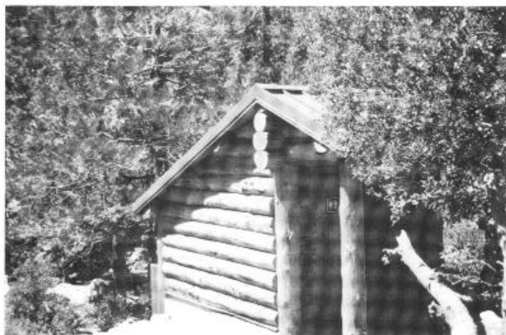
Figure 16. Nevada Falls, Yosemite National Park. Yosemite site built compost toilet basement is fully insulated. Intake air is pulled through a heat collector on the roof.
