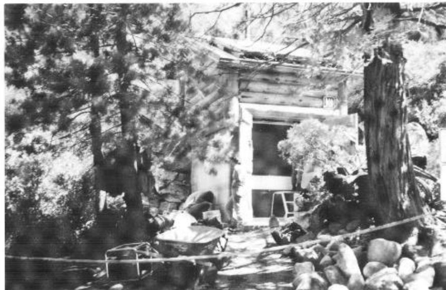
Figure 43. Yosemite National Park Site-built Composting Toilet, basement. The daylight basement has double doors that open to increase the maintenance space.
