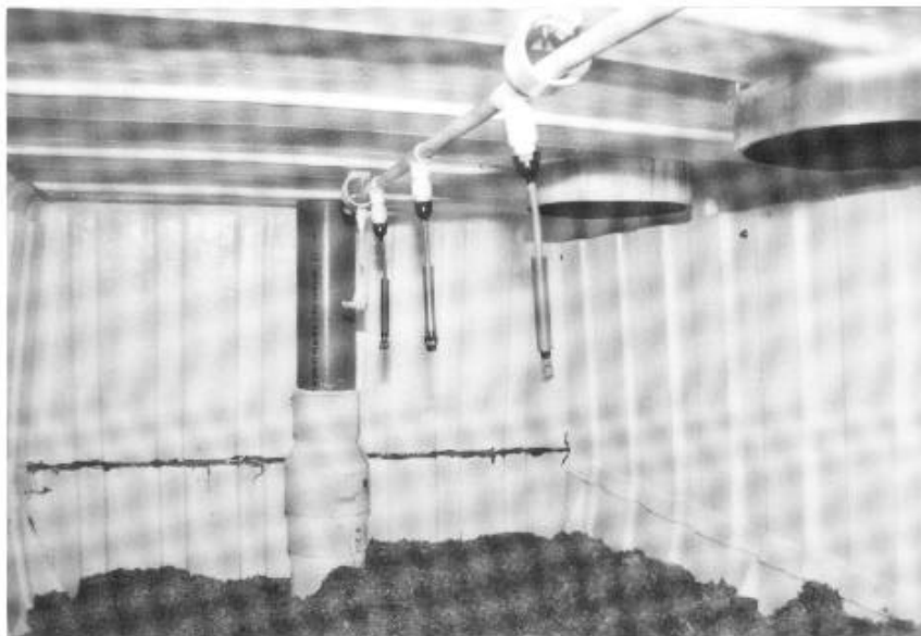
Figure 23. Internal fresh water spray system standard on DEVAP™ 2000 tank by Biological Mediation Systems, Inc. (BMSI).
