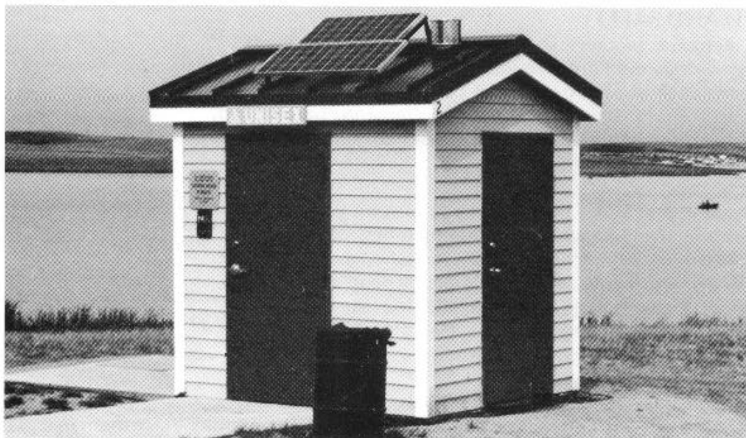
Figure 21. This building is located on flat ground and has restricted basement access, but all components of the electrical and ventilation system are serviceable without entering the basement. Building by BMS.
