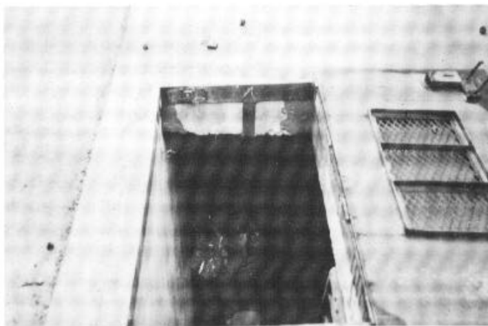
Figure 4. Hatches make maintenance difficult. They also result in confined space areas.
