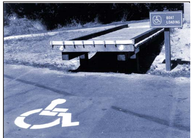
Figure 10—Reflectors are recommended for loading platforms.
