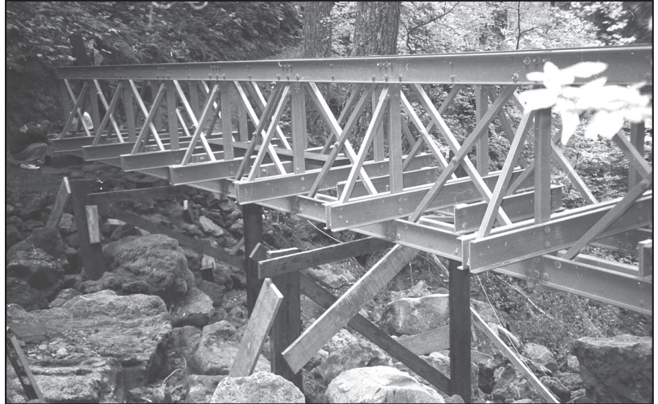
Materials for this fiber-reinforced polymer bridge weighed just 4,000 pounds rather than 10,000 pounds for a comparable steel bridge.
